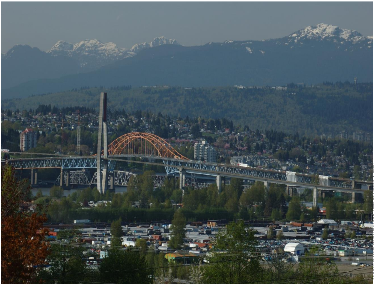
Bridgeview Industrial Park and Pattullo Bridge, Surrey.
