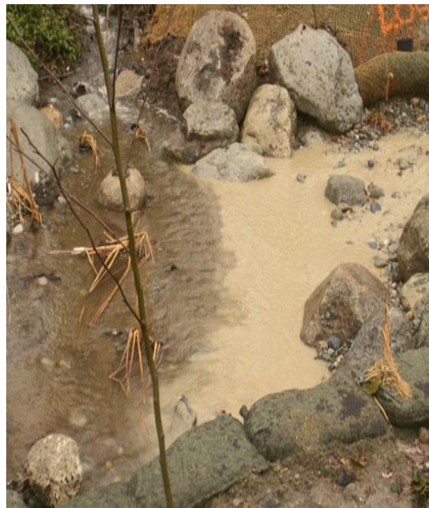
Sediment from poor site development practices.
