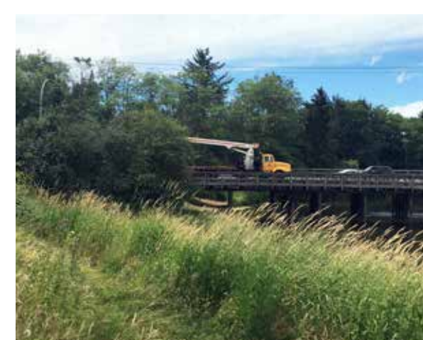
Bailey Bridge / King George Blvd Crossing
