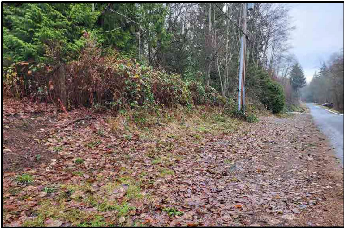
Photograph B10. East view of 92 Avenue, taken from the driveway of the western property; note no ditch is present (December 13, 2022).
