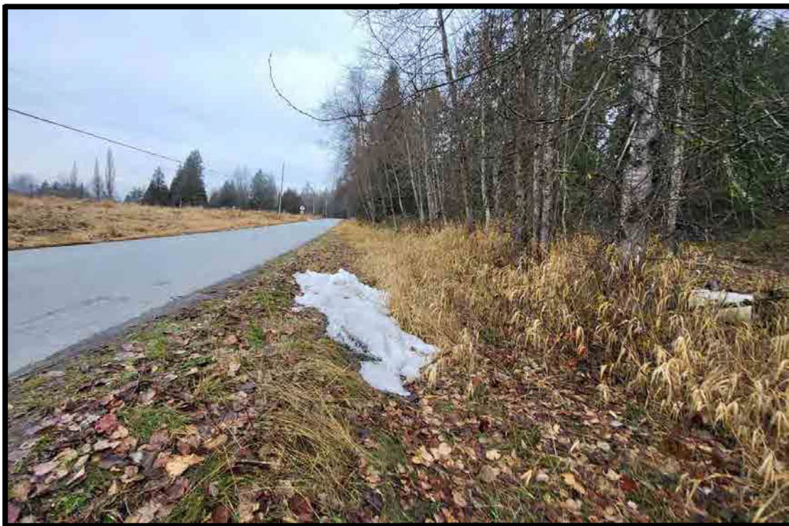
Photograph B16. North view of Bothwell Drive, taken near a vehicle access point to the western property; note there is no defined ditch (December 13, 2022).
