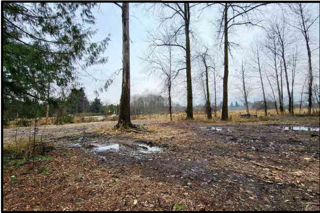
Photograph B17. Southwest view of saturated lands in the southwest corner of the property, taken near the toe of slope (December 13, 2022).
