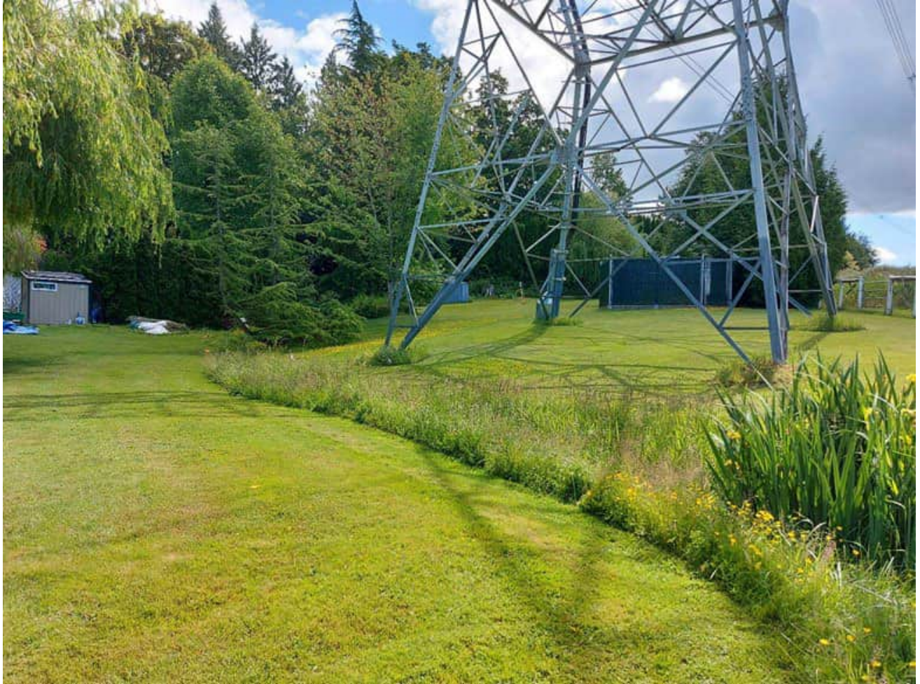
Photograph 5. View of WC2 facing east. WC2 flows within the longer grassed area (Photo taken June 9, 2021).
