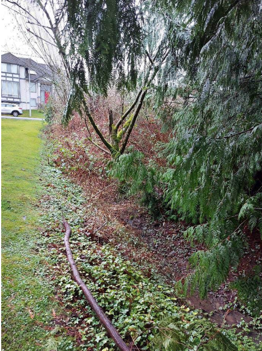
Photograph 1. View of Ditch 1, north of the subject property facing east. The ditch was conveying marginal flows even during a significant rainfall event. (Photo taken February 1, 2021).
