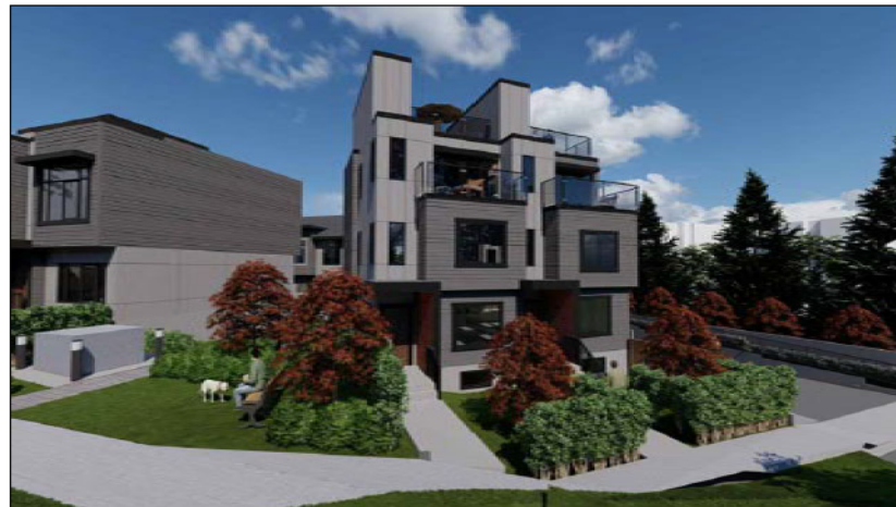
STREETVIEW FROM PARKWAY DRIVE (NORTH ELEVATION - BUILDING 7)
