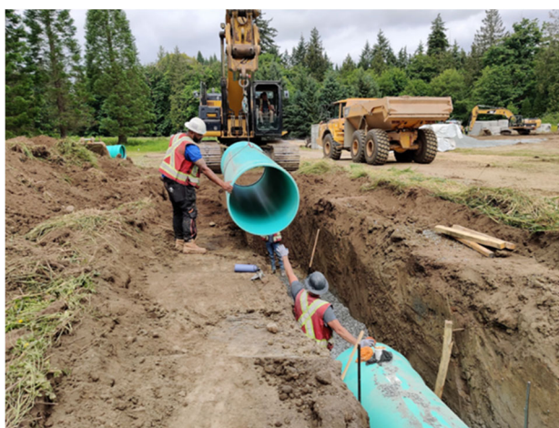
Twin Trunk Sewer Construction on Tynehead Trunk Sewer in Fleetwood
