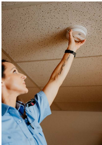
Firefighter checking a smoke alarm
