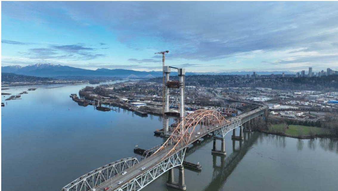
Pattullo Bridge Construction
