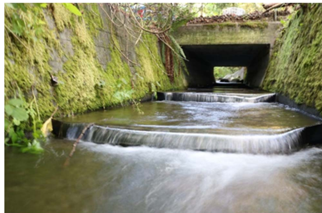
Flexi Baffle Installation on Bon Accord Creek
