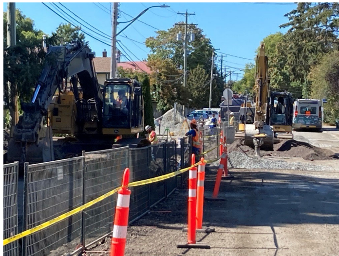
Engineering team on site in Surrey
