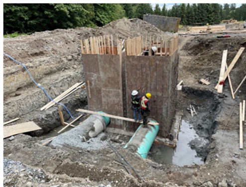
Construction of Sewer Chamber for Tynehead Twin Sewer
