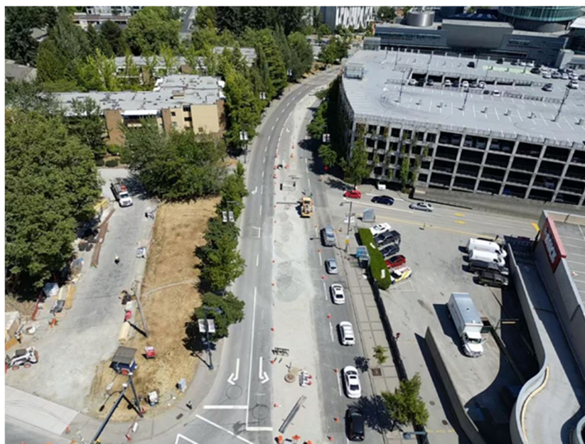
Trunk Sewer Construction on University Boulevard near Old Yale Road
