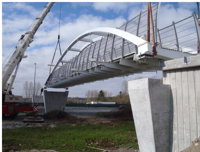
Pedestrian Over cross Construction
