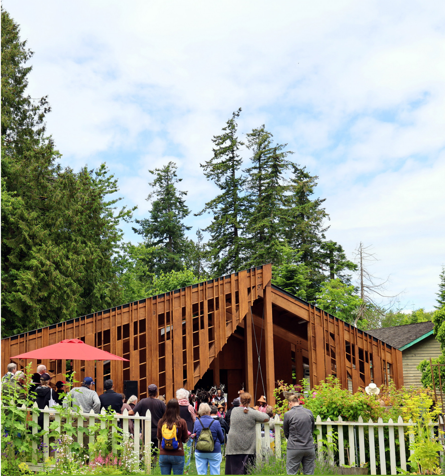
Completed the construction of Totest Aleng: Indigenous Learning House
