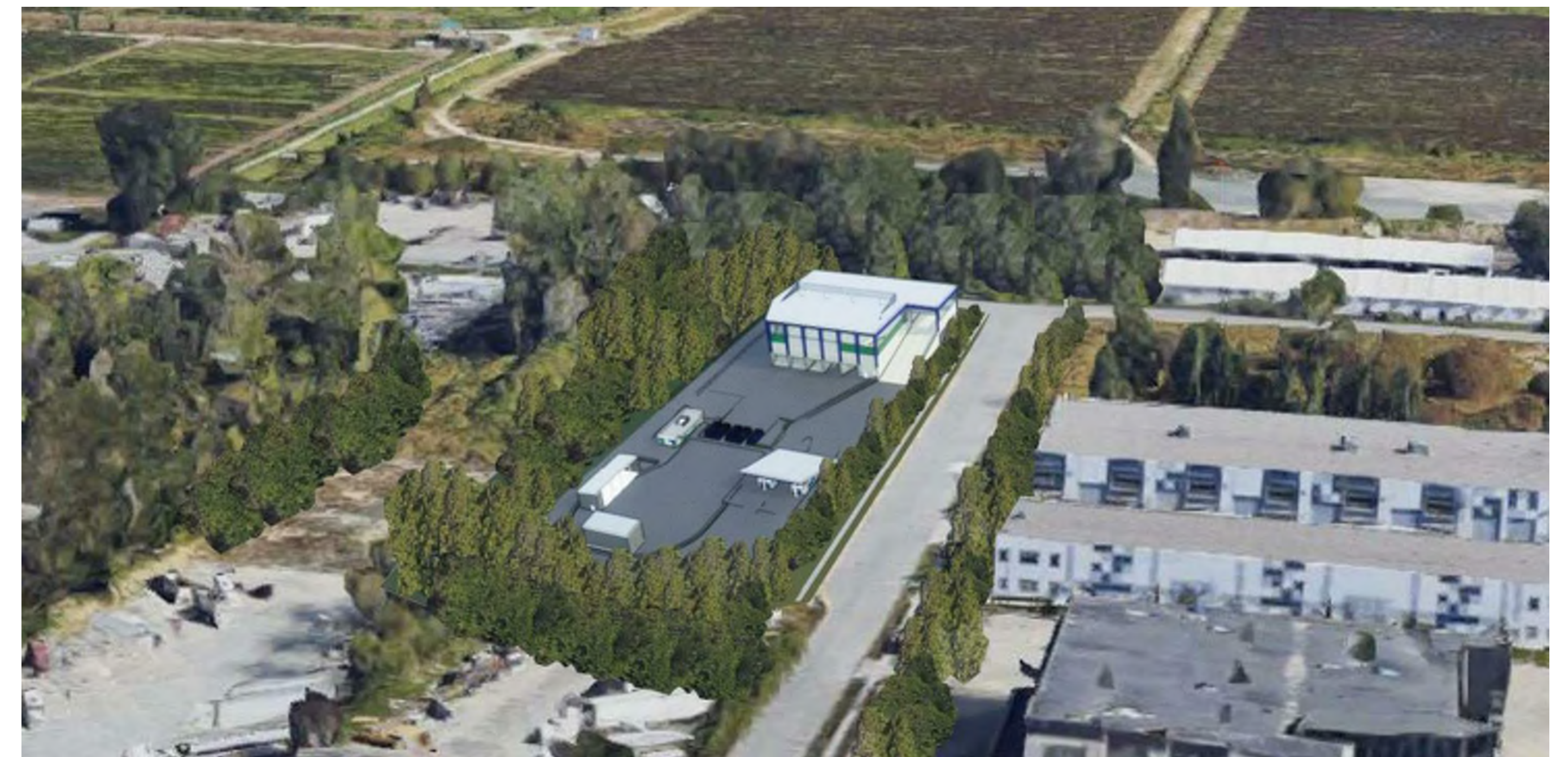
SOUTH WEST AERIAL VIEW
