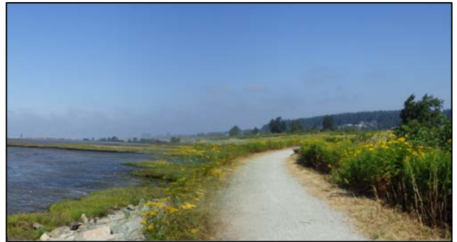
Colebrook Dyke Existing Crest
