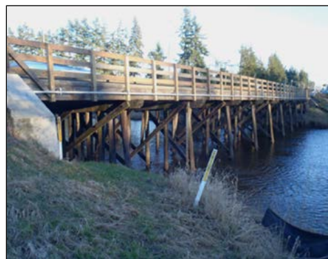
Existing Nicomekl Bridge
