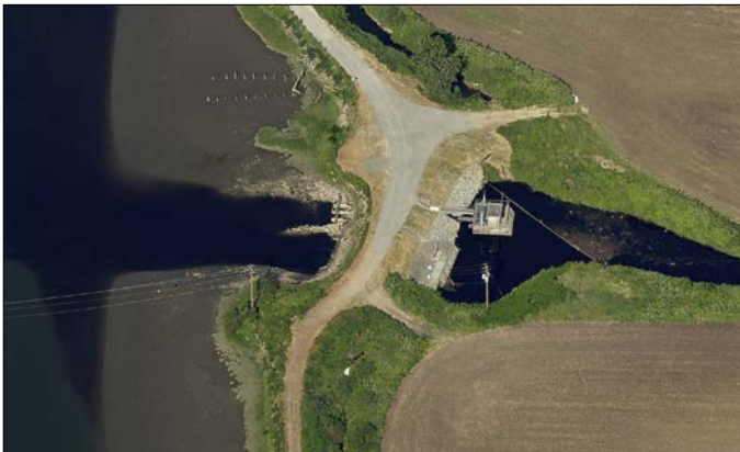
Existing Colebrook Drainage Pump Station
