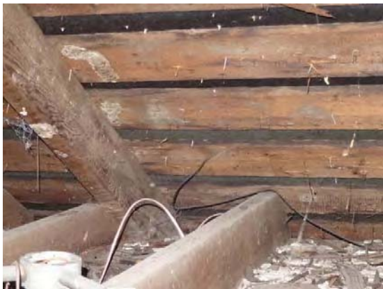
One rare occurrence of rafter coinciding with ceiling joist.
