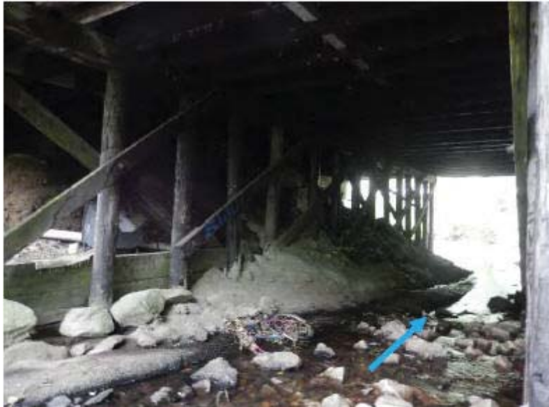
Photos of the Existing Timber Trestle Bridge
