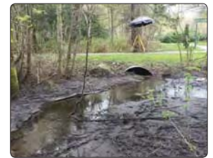
CULVERT IN BON ACCORD CREEK
