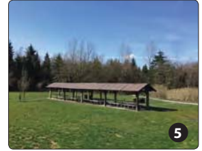
PICNIC SHELTER AREA
