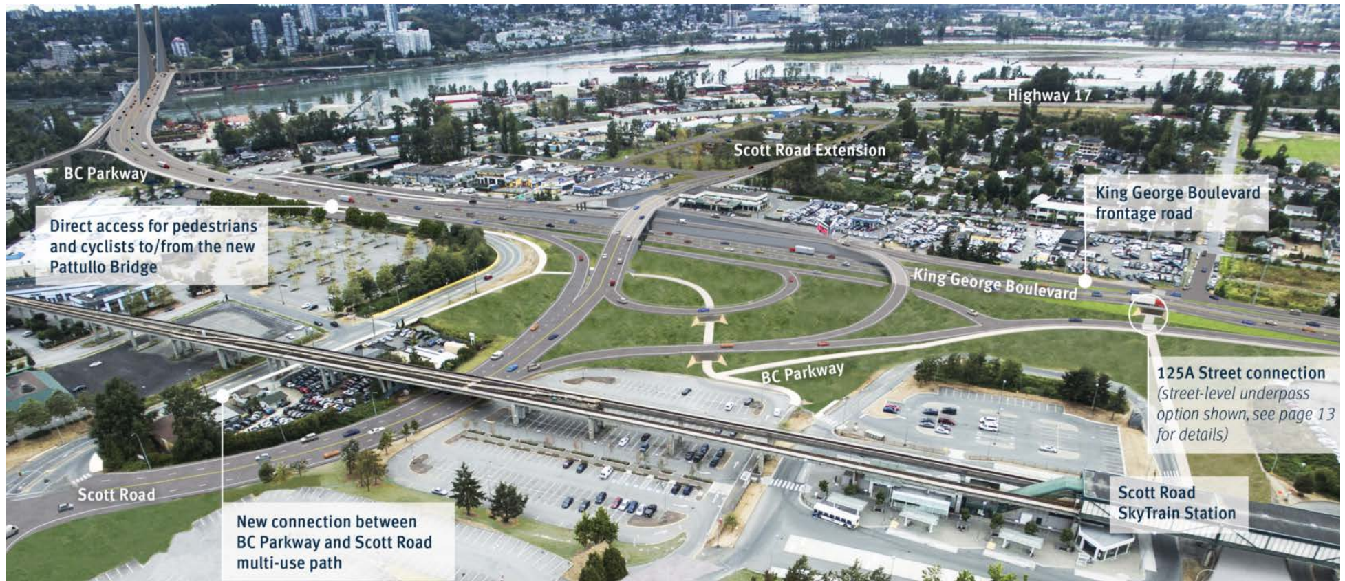
Source: Pattullo Bridge Replacement Project Community Connections Phase 2 Consultation: Discussion Guide and Feedback Form October 3 – October 31, 2016
