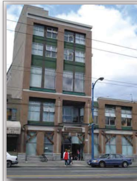
Crabtree Corner & Sheway 533 East Hastings, Vancouver
