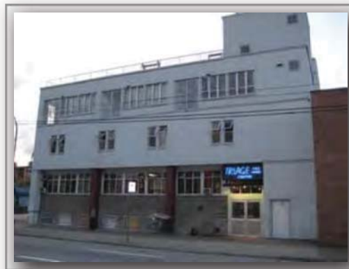
Triage Shelter & Windchimes Housing Source: raincityhousing.org
