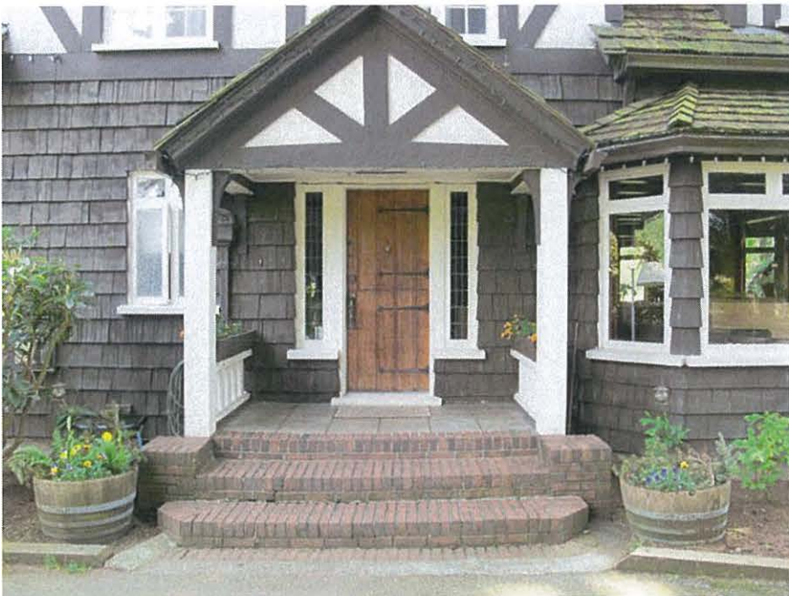
Front Entryway, West Façade
