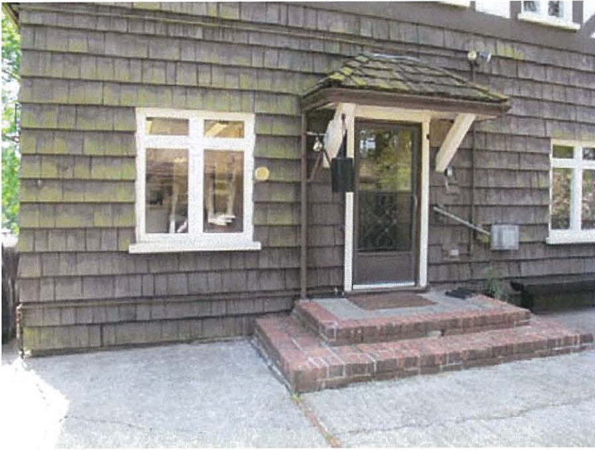
Side Entryway, North Façade
