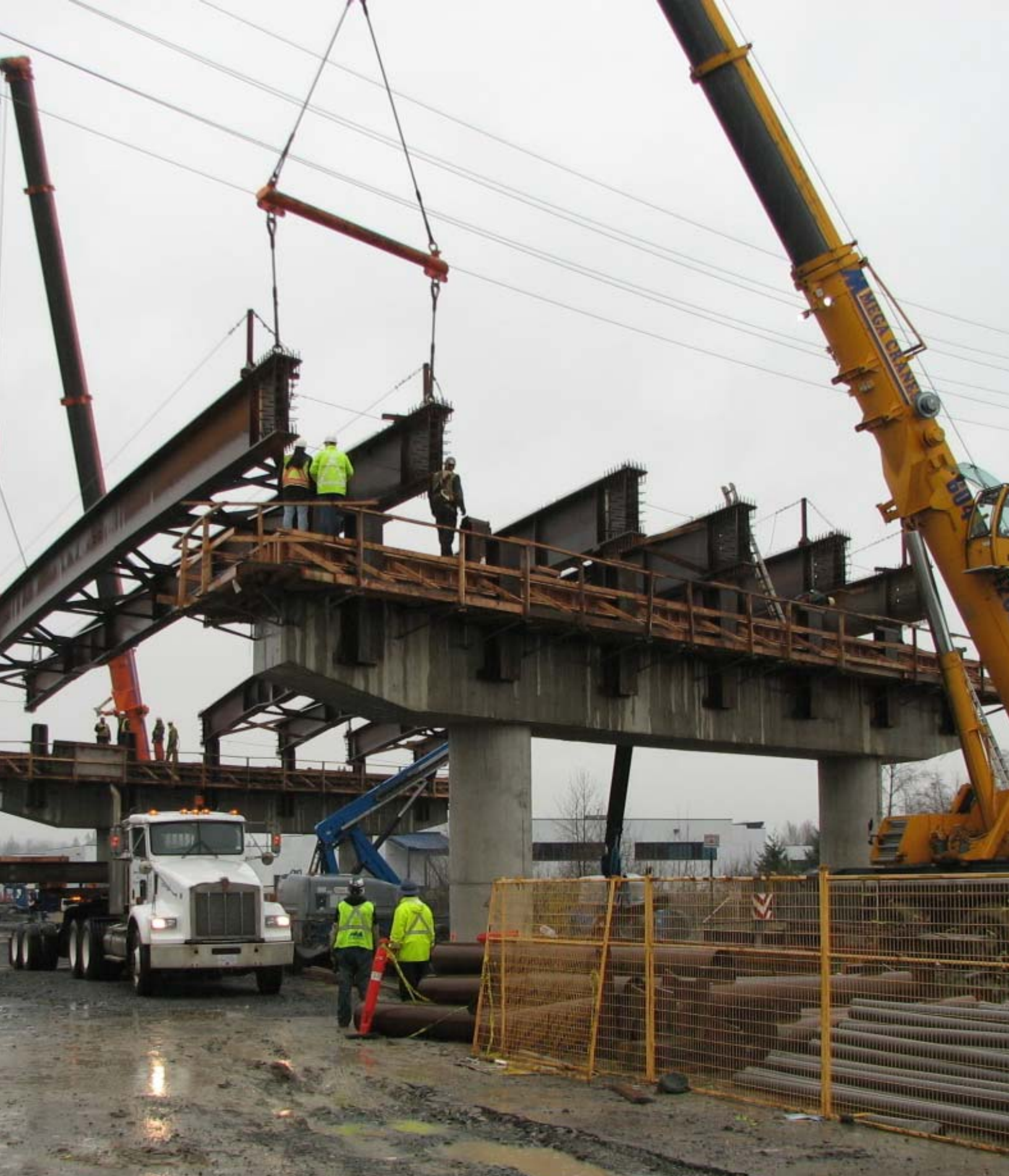
196 Street Rail Overpass
