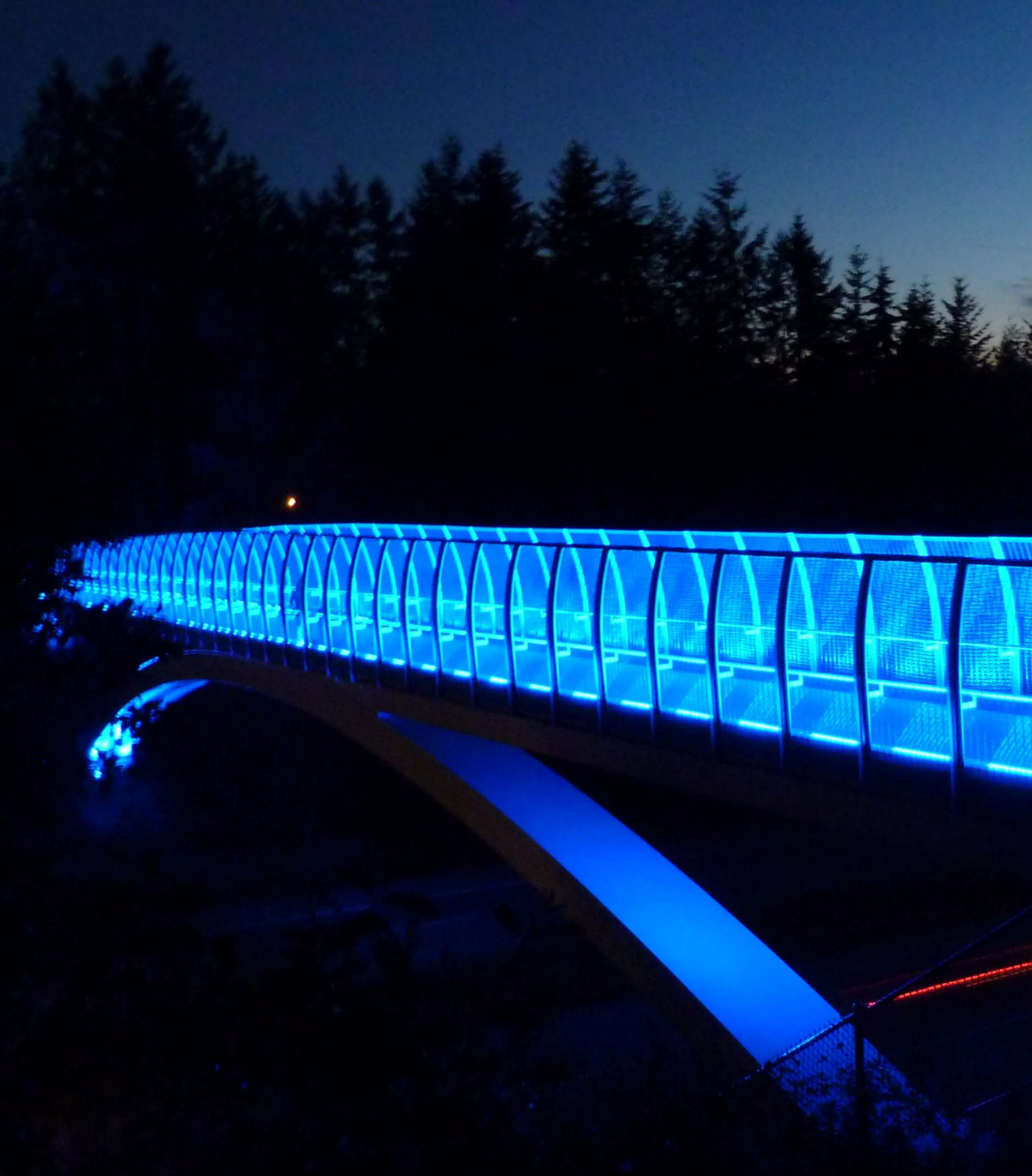
Highway 99 Pedestrian Overpass
