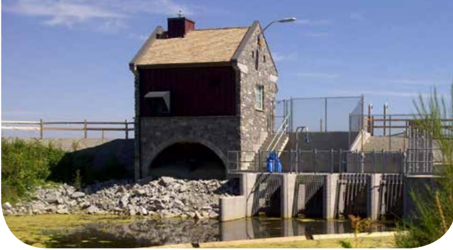
The new Maple Drainage Pump Station in Crescent Beach improves drainage and reduces the risk of flooding.
