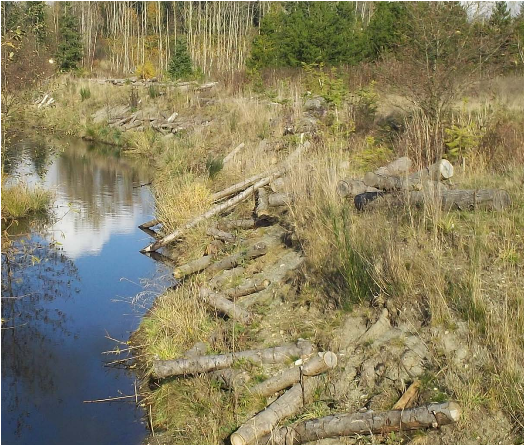
Coarse woody debris placement discourages trail-use and stabilized bank - 2011
