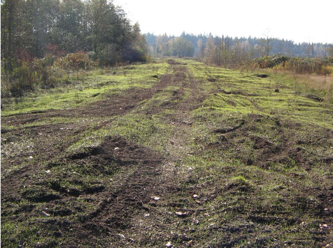
Decommissioned road with 90cm topsoil placed 2009
