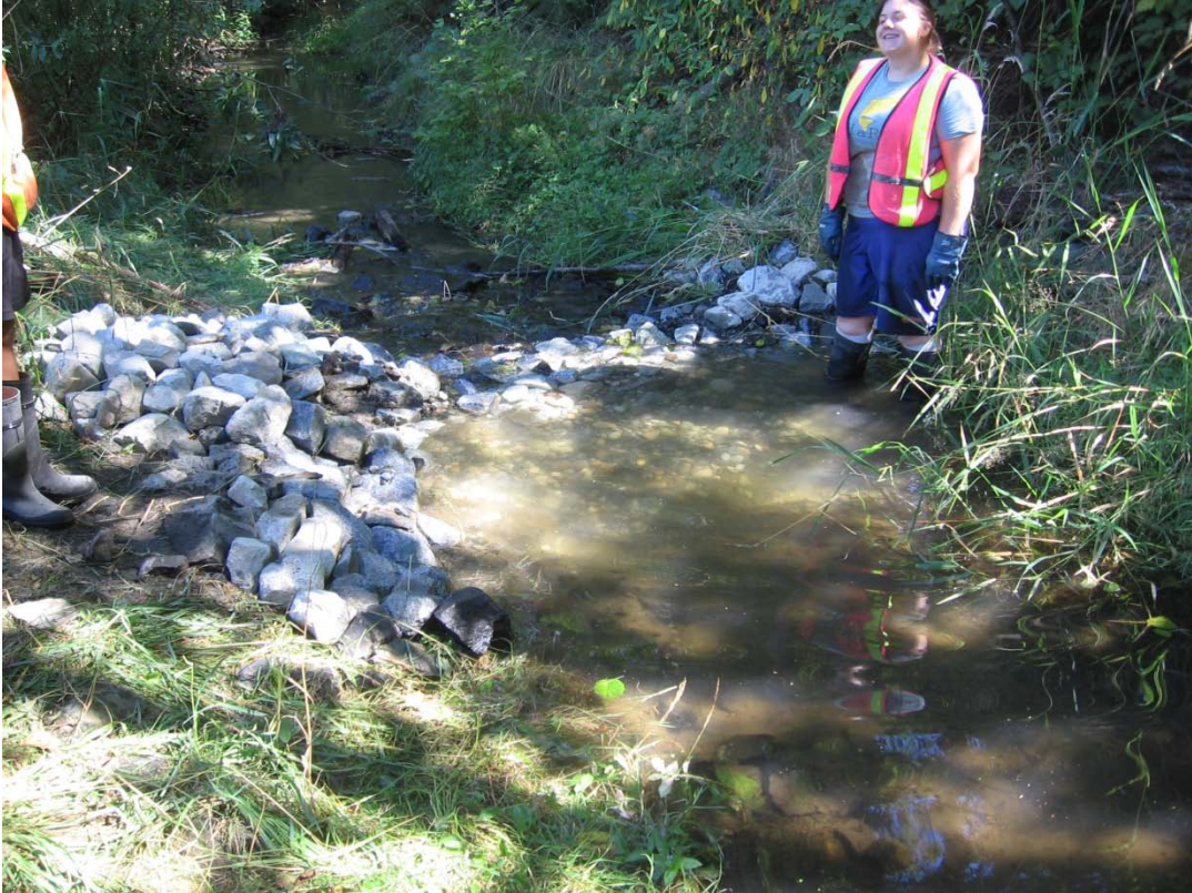
SHaRP students constructing gravel spawning platform - 2011
