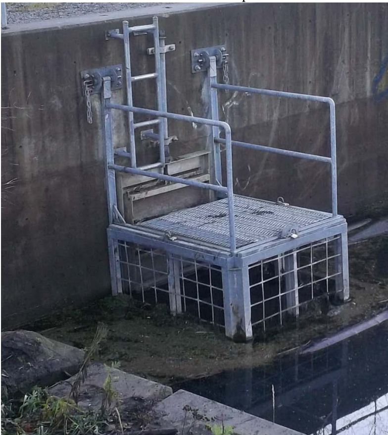
Beaver Deceiver installed at detention pond control structure
