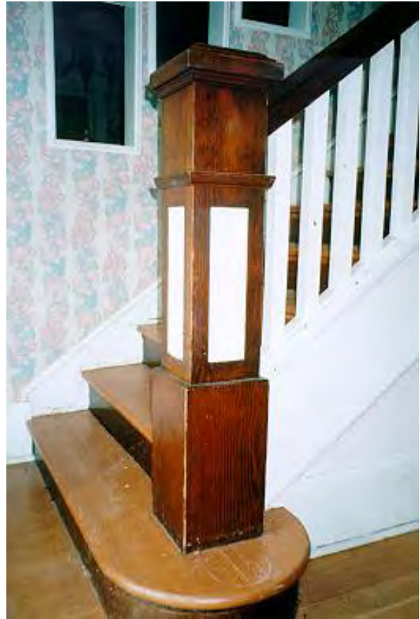
Details of staircase woodwork, including newel post and newel cap.
