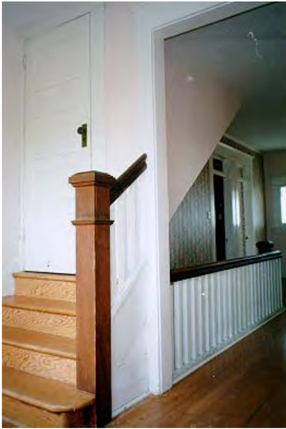
Stairs leading to third floor, with a plain newel post.
