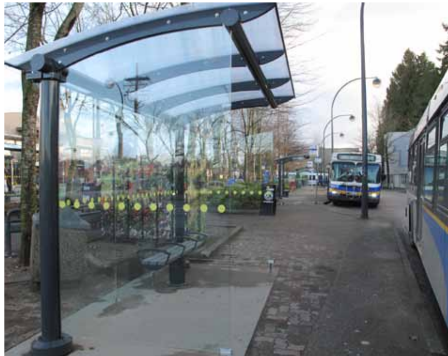
New bus shelters at Newton Bus Loop.
