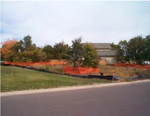
Tree Protection Fences in Place during Construction
