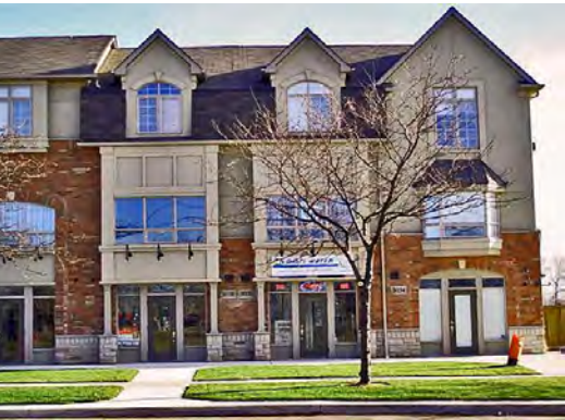
Row Housing containing ground floor retail and office space
