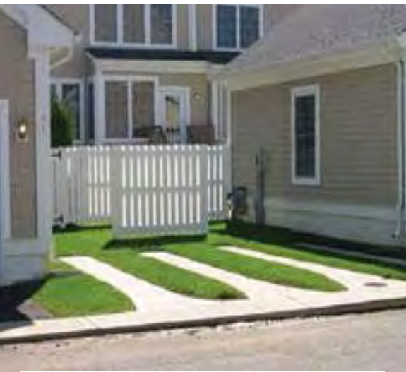
Wheel strips provide a stable base for vehicles; an unpaved driveway allows for increased infiltration.
