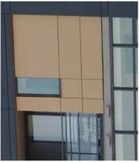
HORIZONTAL PANEL ON EXTERIOR FACADE
