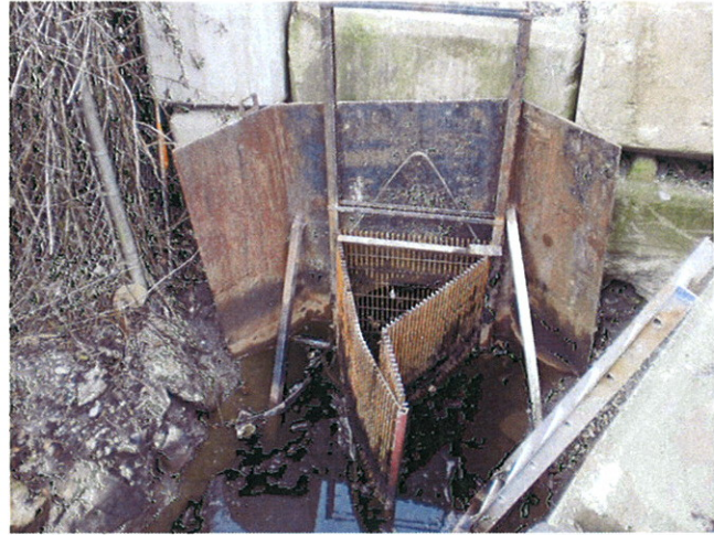
Photo 2: Culvert headwall at southeast corner of #11678 130 th Street.
