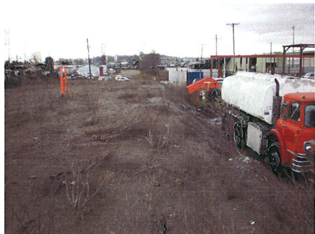
Photo 4: Photo from top of South Fraser Perimeter Road preload looking west along 11678 130 th Street property line.
