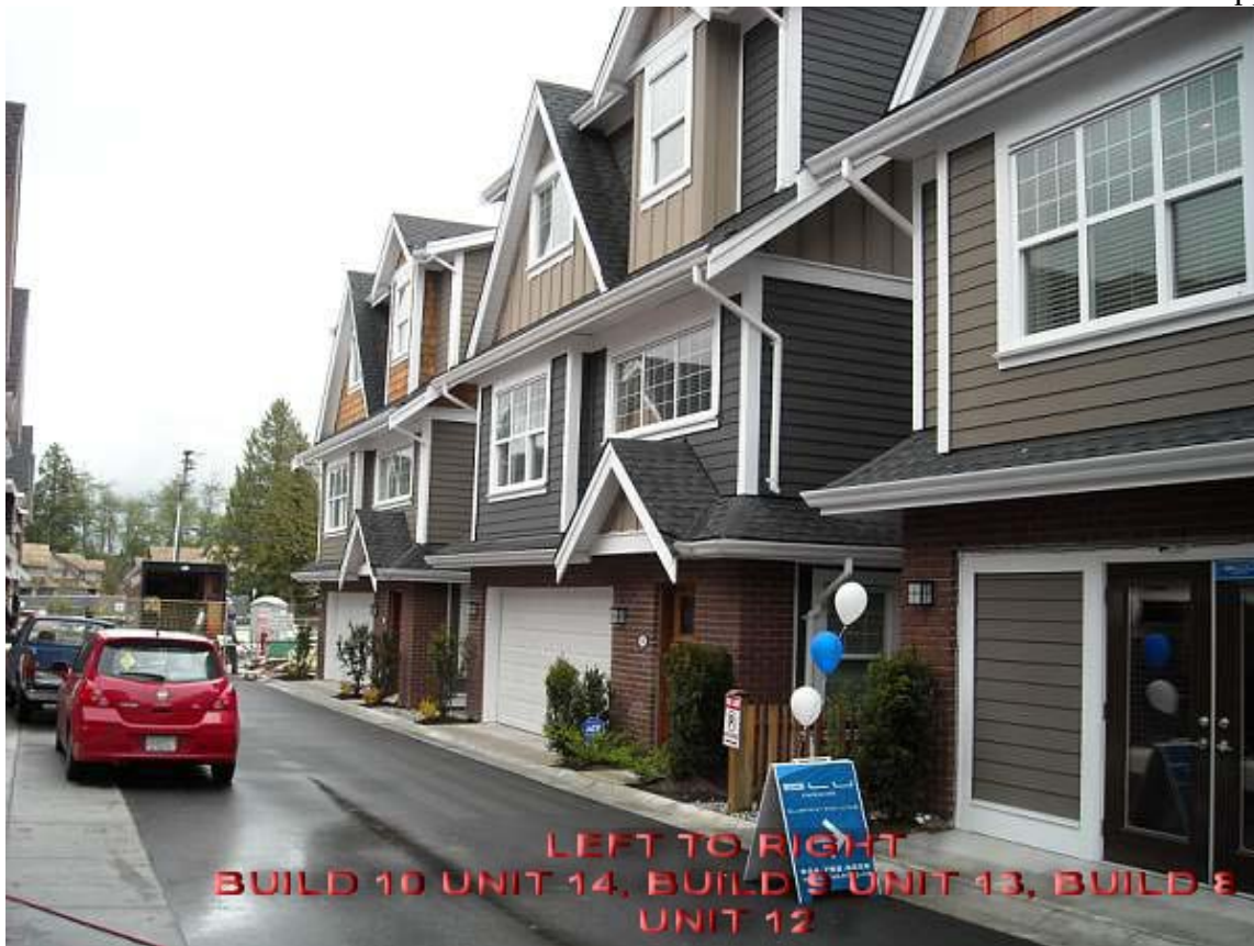
Left to Right – Building 10 Unit 14, Building 8, Unit 13, Building 8, Unit 12
