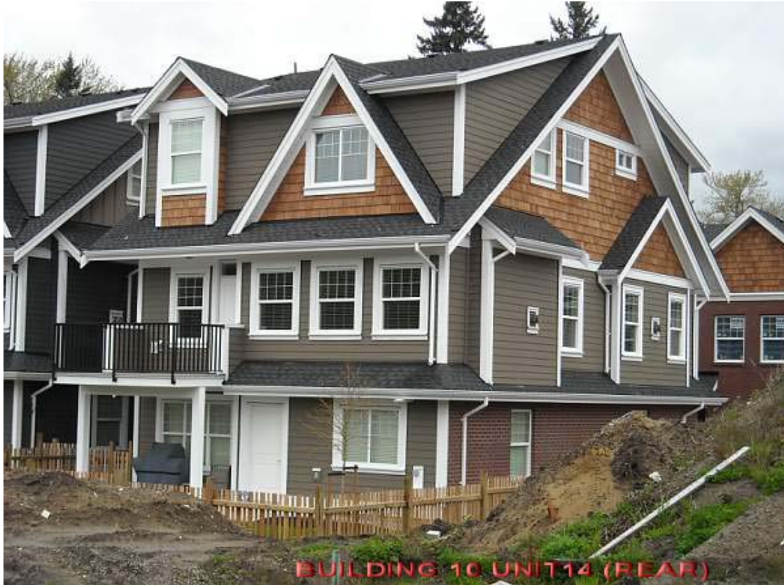
Building 10, Unit 14 (rear)
