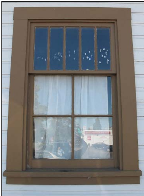
5-over-4 multi-paned double-hung wooden sash windows - north elevation
