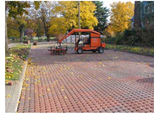
Ecolock Pavers curb-to-curb
