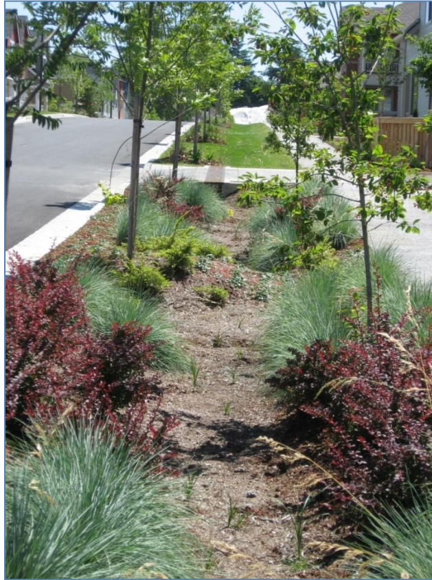
Landscaped Bioswale, High Point Development, Seattle, Washington
