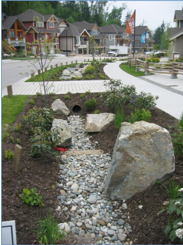
Bioswale, Maple Ridge, BC
