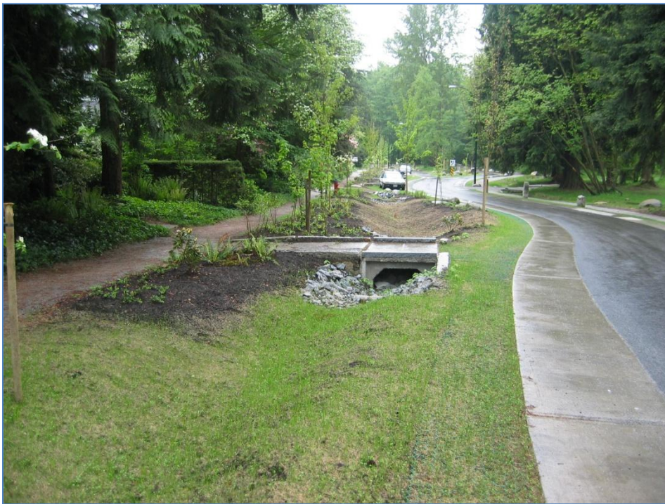
Grassed Bioswale, Crown Street, Vancouver, BC (Note access across swale at center of photo)
