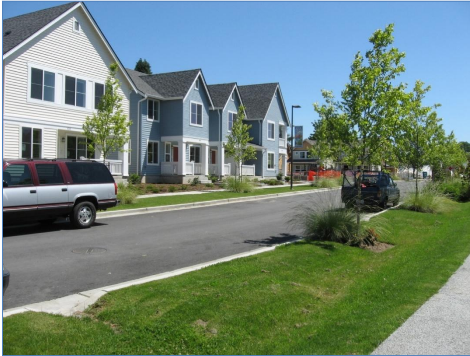
Grassed Bioswale, High Point Development, Seattle, Washington (Note curb drop to allow runoff to enter swale from street, in lower left of photo)
