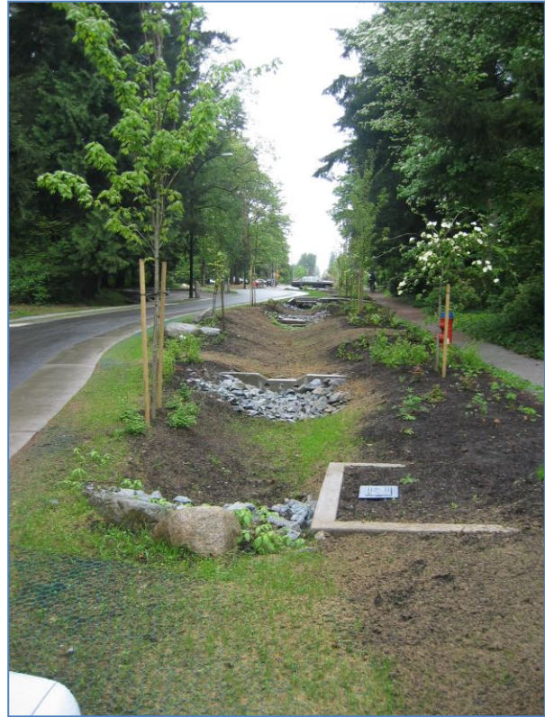
Bioswale with grade control structures Crown Street, Vancouver, BC
