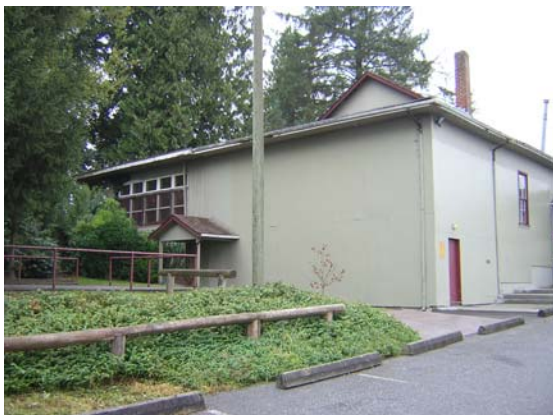
View of the rear showing the eastward extension to the Hall.
