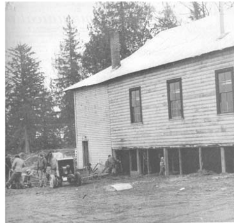
A photograph of the basement being added in the 1970s.
