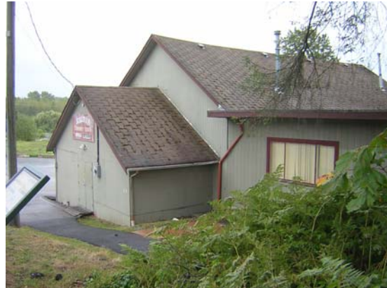
View from the south west showing the front of the building, the storyboard installed along 152 Street and the addition to on the south side of the Hall.
