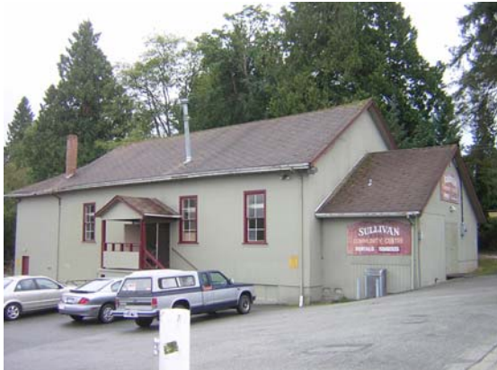
View of Hall from north west, showing the current entrance at the side of the building.
