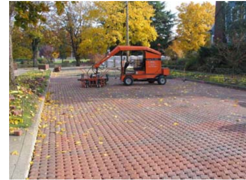
Ecolock Pavers curb-to-curb SE Knapp St. from 21 st to 22 nd Ave.
