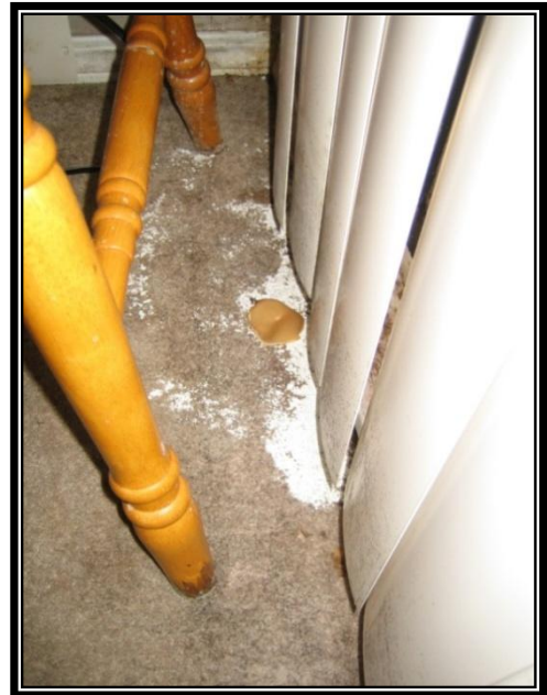
Fungus and mould cover the carpet in one unit.
