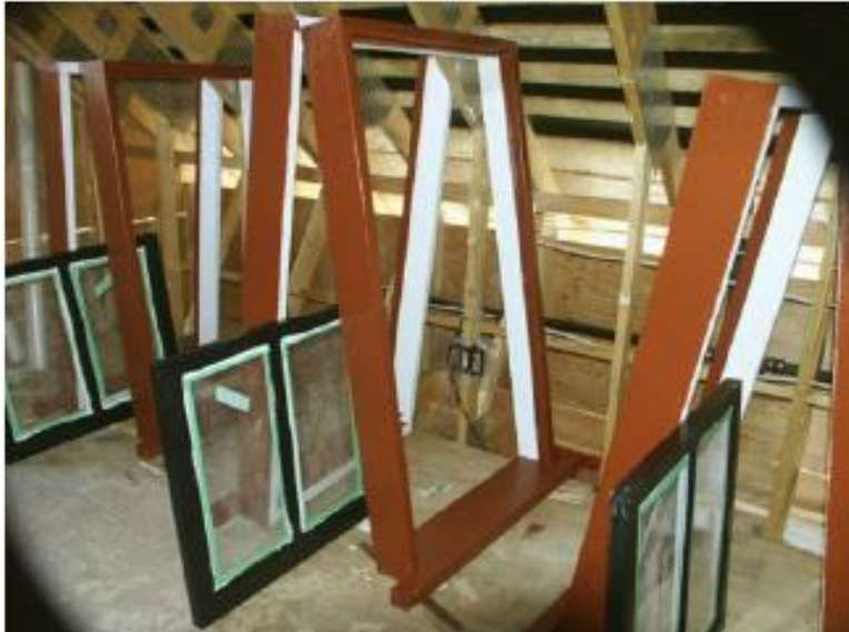
A view of replica cedar window frames and rehabilitated existing sash.
