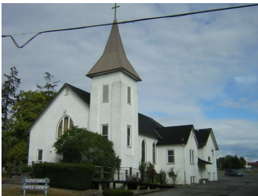
View of church and bell tower.
