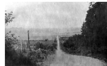
View south along Coast Meridian Road in earlier years would be similar to that for Old McLellan Road
