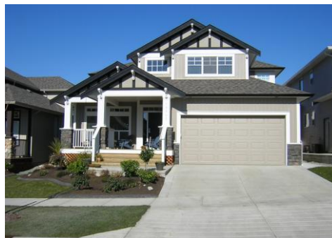
House with stair consisting 3 risers in the setback
