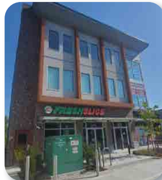
New Office Building
