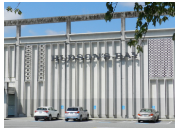
Former Woodward's Building
