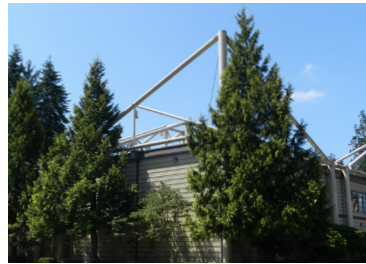
Former Expo '86 Pavilion
