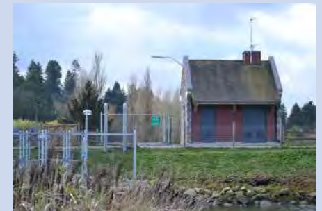
Maintain flood infrastructure: pump stations
