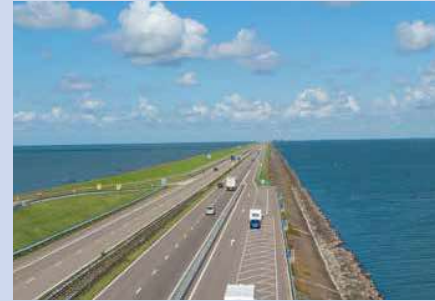
Raised highway becomes flood barrier.
