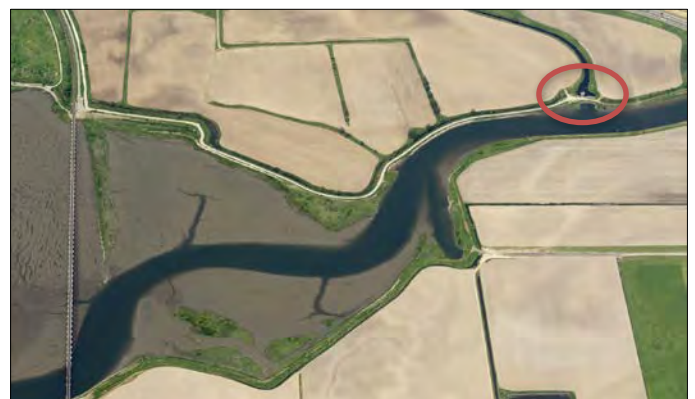
Mouth of the Serpentine River with Colebrook Drainage Pump Station (view from south)
