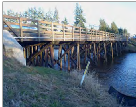
Existing Nicomekl Bridge
