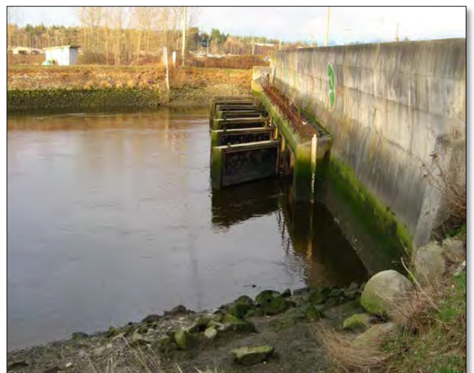
Serpentine Sea Dam at low tide with gates open
