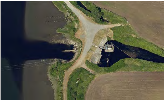
Existing Colebrook Drainage Pump Station
