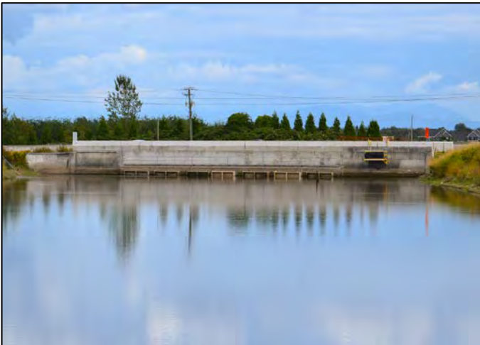
Serpentine Sea Dam at high tide with gates closed
