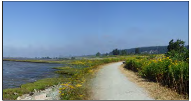
Colebrook Dyke Existing Crest
