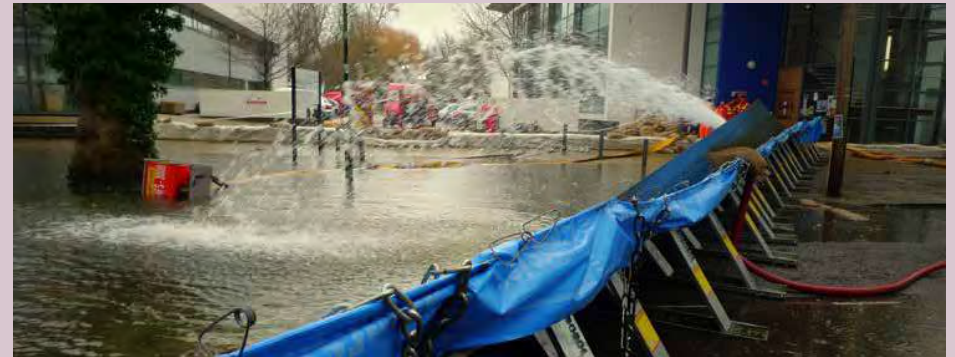
Temporary flood walls in the UK CC-by-sa, Henry Burrows, flickr.com
