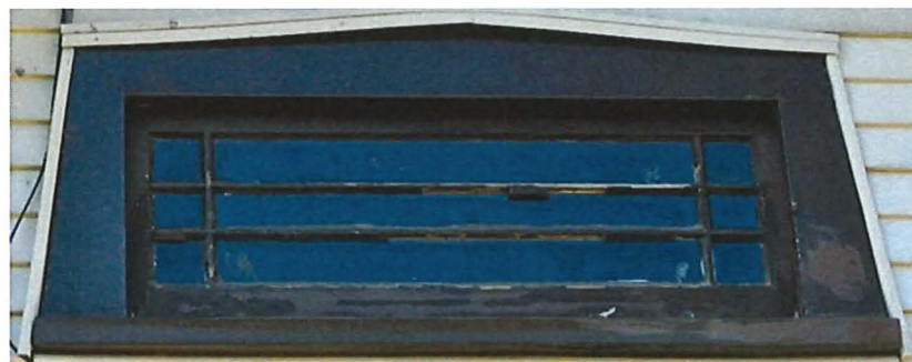
Figure 37: : Attic window A-02
