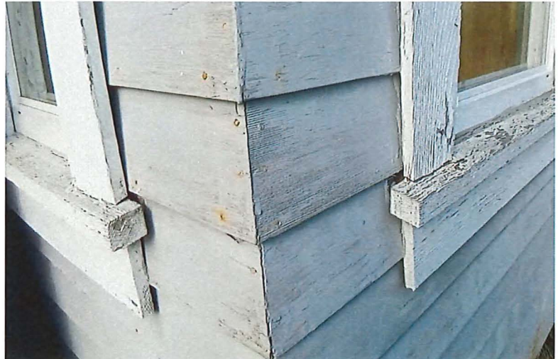
Figure 78: Tapered siding corner
