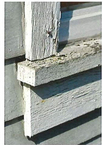
Figure 85: Bottom plate and sill end
