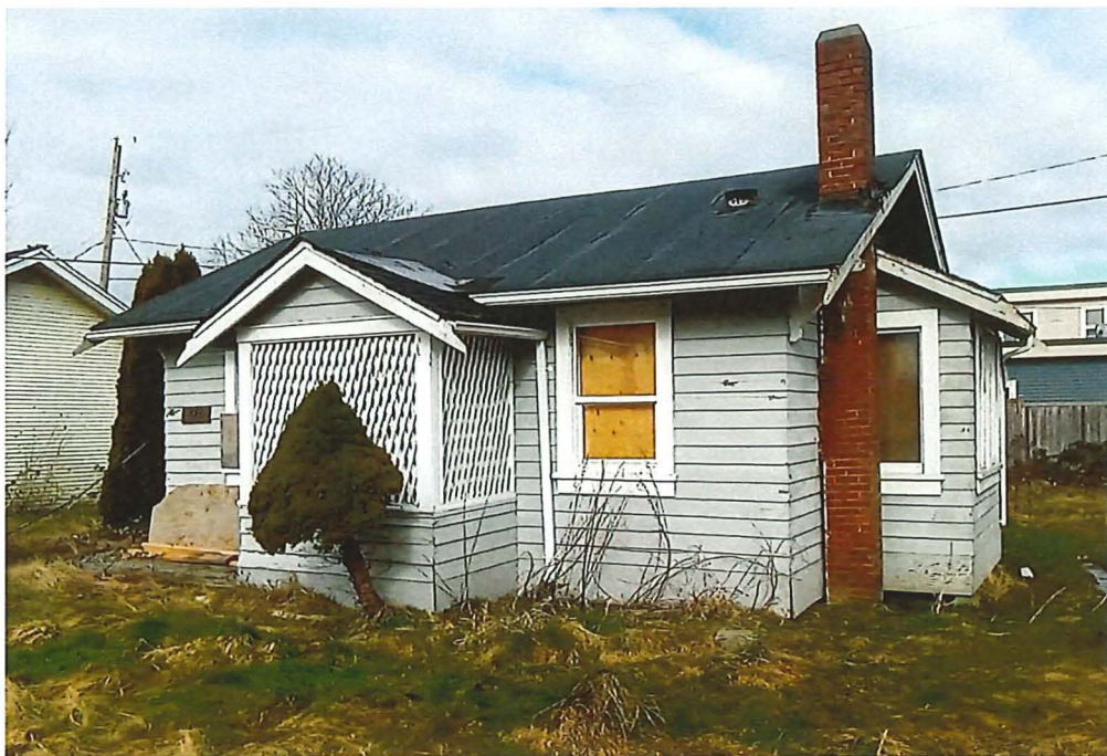
Figure 62: Northeast corner of the Mooring Cottage
