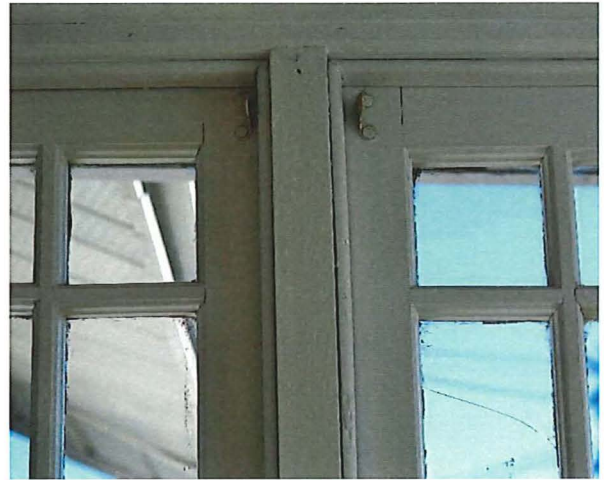
Figure 34: Interior view of W-05
