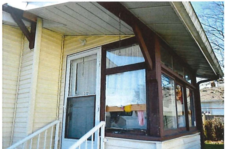
Figure 31: Back porch details of knee bracket, door, and windows
