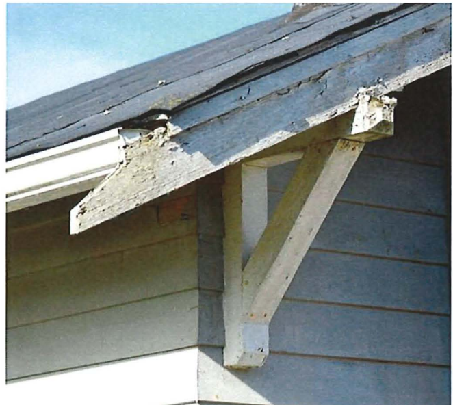
Figure 74: Tar paper roofing, bargeboard, and knee-bracket
