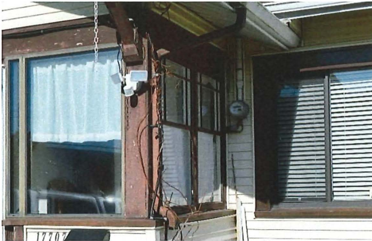
Figure 33: front door with W-03-02-01
