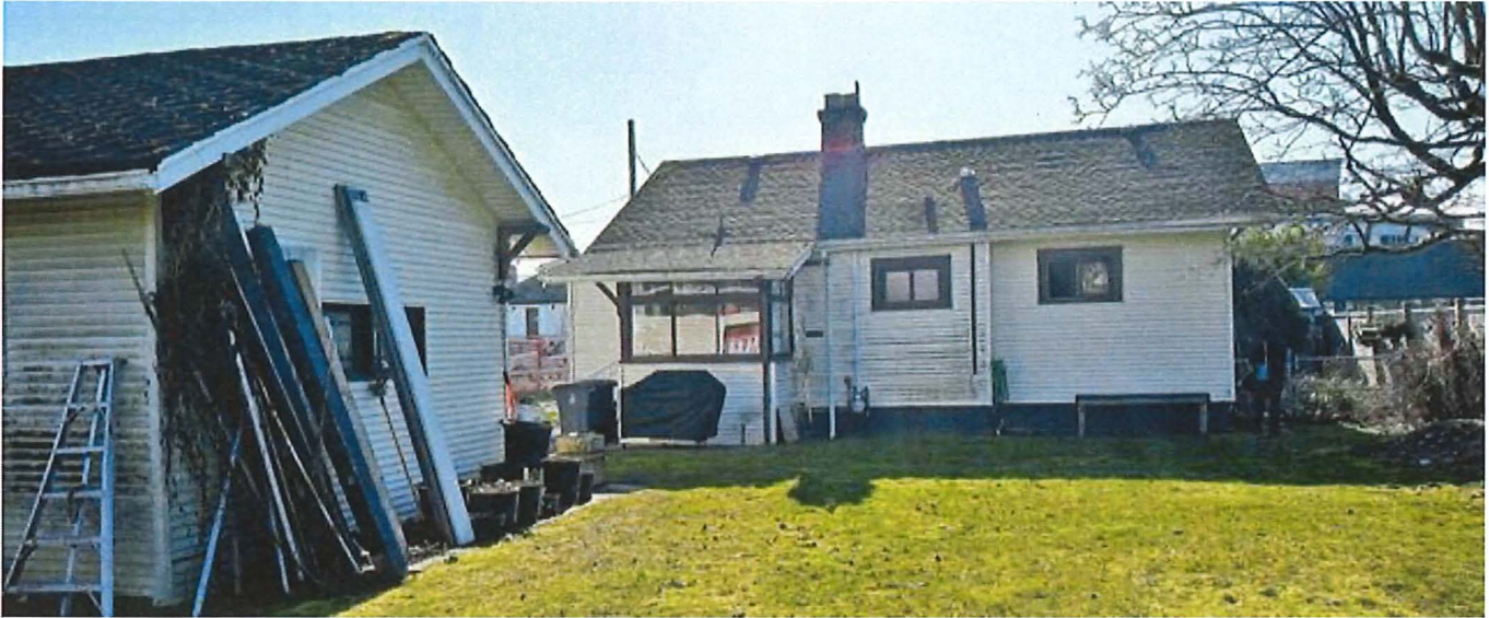
Figure 14: Backyard of the Mooring House with same style garage on the left
