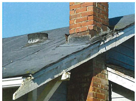
Figure 76: Tar paper roofing and chimney flashing
