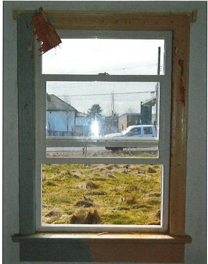
Figure 82: W-02 Interior face of double-hung window
