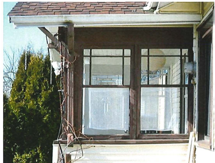
Figure 28: Original side windows of the front porch
