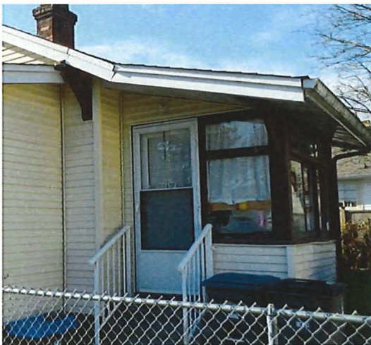
Figure 30: Enclosed back porch with shed roof
