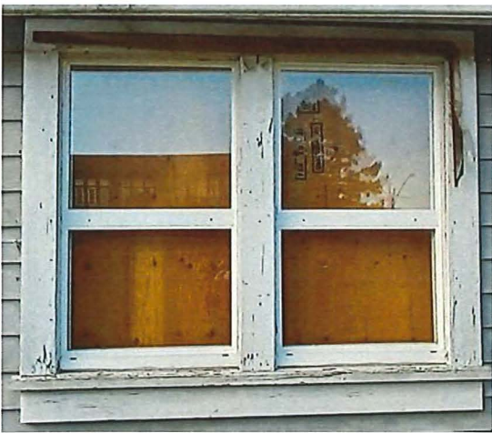
Figure 83: Pair of double-hung windows at dining nook W-07
