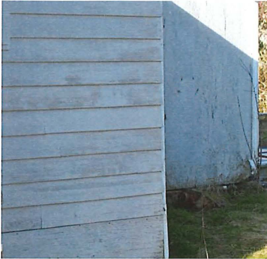
Figure 77: Typical lap siding with plywood addition behind
