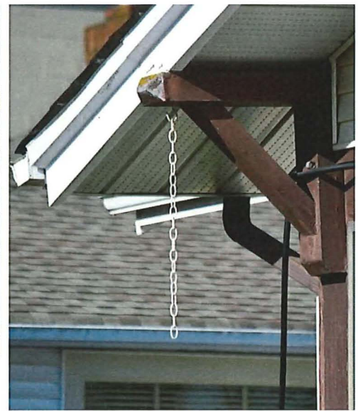
Figure 24: Knee-bracket with pointed end at southwest corner of front porch
