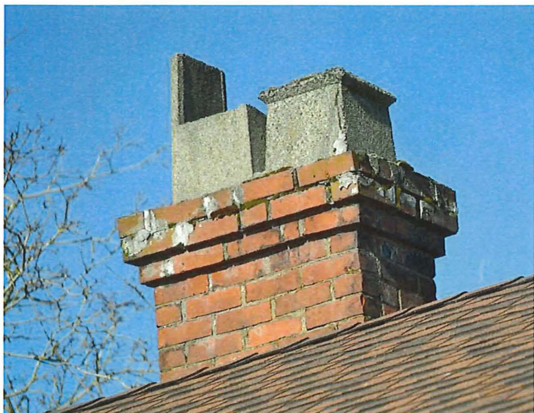
Figure 52: Exposed chimney shaft viewed from 56A Avenue
