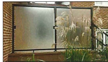
PONDER COATED ALUMINUM PRIVACY SCREENS BLACK ALUMINUM WITH OBSCURED TEMPERED GLAZING ELEVATIONS FINISH SCHEDULE NO. 10
