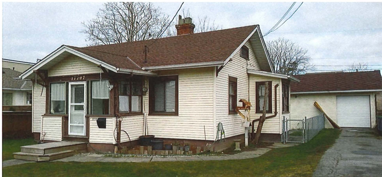
Figure 9: The Mooring House view of northeast corner with the garage at the back
