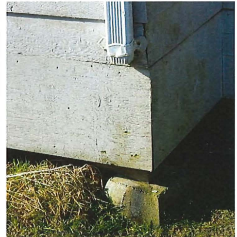
Figure 70: plywood base board and block footing
