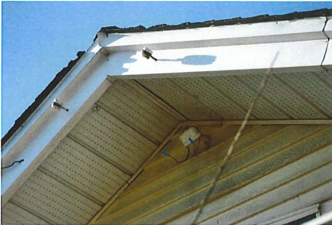
Figure 20: Gable end with closed perforated aluminum soffit
