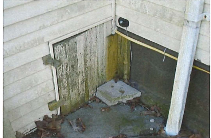
Figure 17: Crawl space access half door
