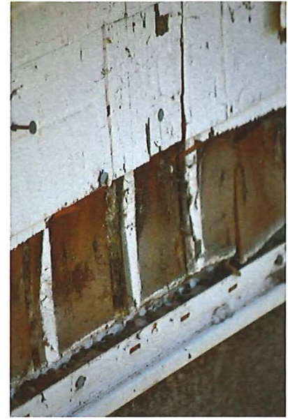
Figure 26: Detail of shingles
