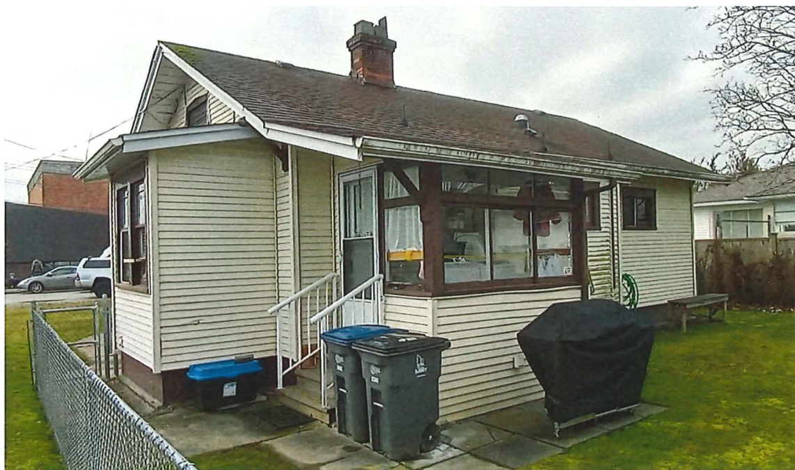
Figure 10: The Mooring House view of southwest corner with enclosed back porch and kitchen/dining nook
