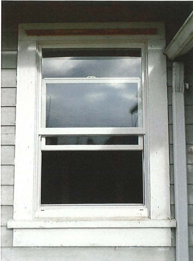
Figure 81: W-02 Front of cottage double-hung window
