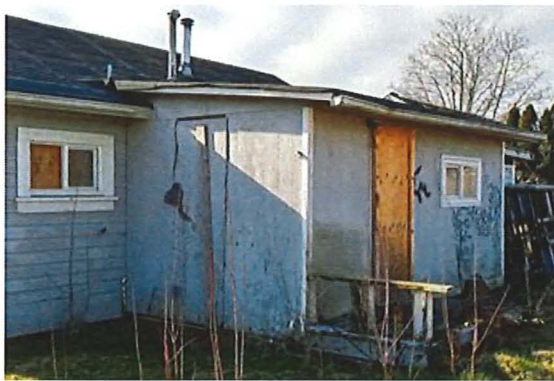
Figure 64: Plywood addition on the back of the cottage
