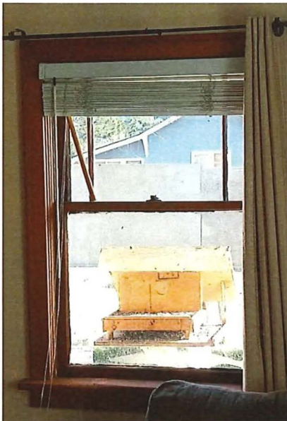
Figure 41: W-11 interior view
