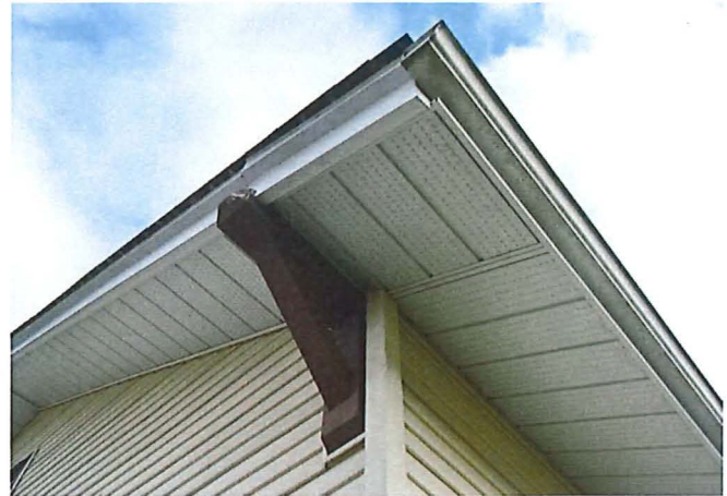
Figure 21: Wooden knee bracket northeastern roof corner
