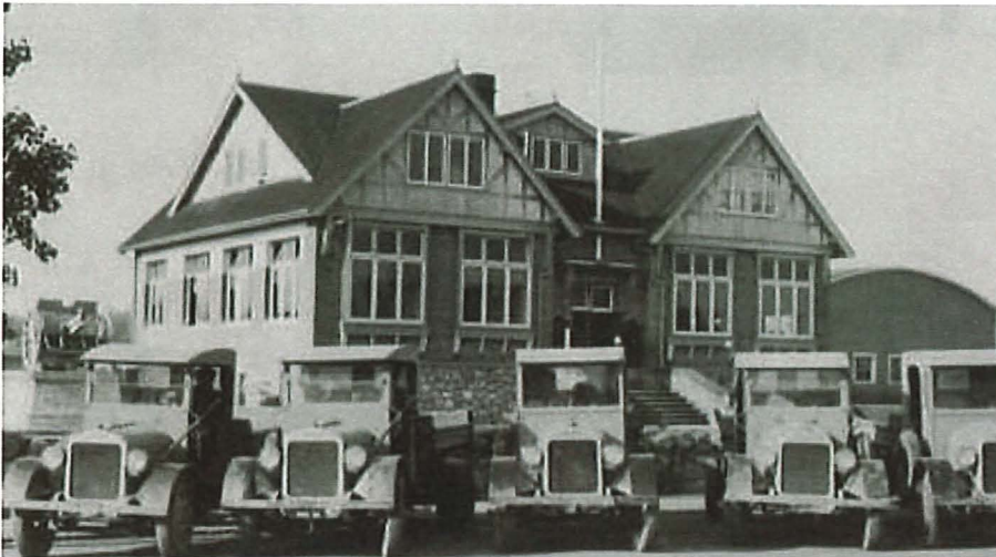
Figure 2: 1912 Municipal Hall, one block south of the Mooring house & Cottage (Surrey Archives)
