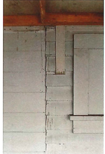
Figure 92: Change of siding on west wall
