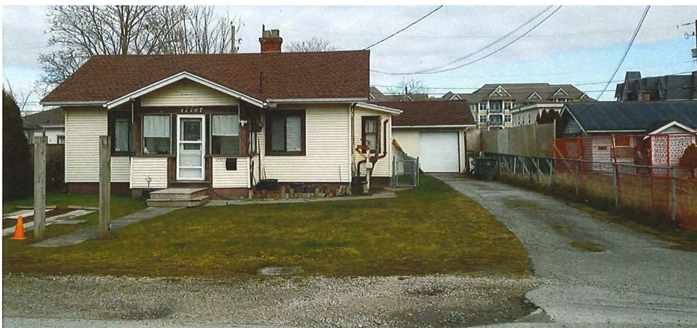
Figure 13: Front lawn of the Mooring House with the garage at the back and the Mooring Cottage next door on the right
