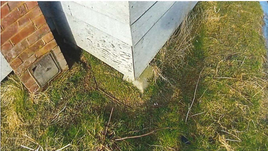
Figure 69: Concrete block footing next to chimney foundation
