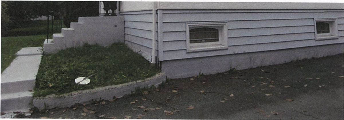
Top: Northeast elevation; Bottom: Foundation at basement level
