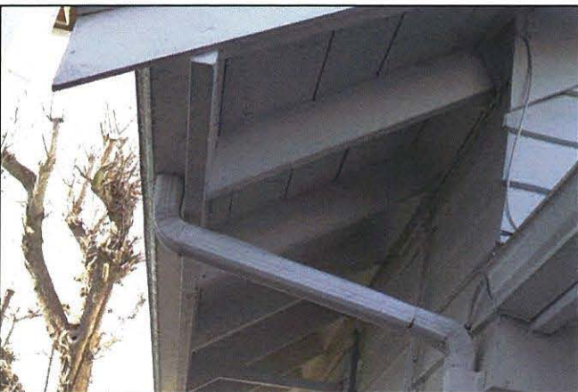
Photo 26: Typ. roof eave, note exposed rafter tails.
