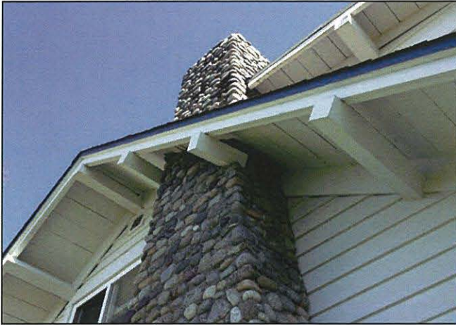
Photo 24: Detail view chimney & roof overhang, note overhang of 1963 dormer.
