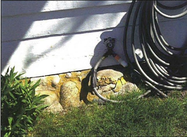
Photo 13: Original stone foundation. Note typical lichen growth.
