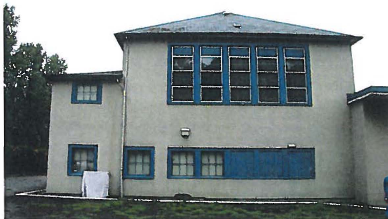
Tynehead School south façade, boarded fenestration replaced with later glazing units.
