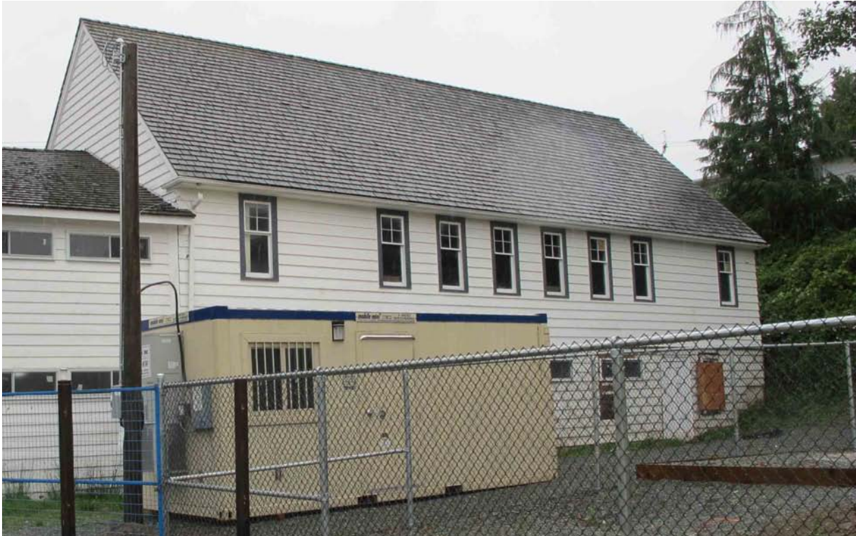
Cedar shingles on roof
