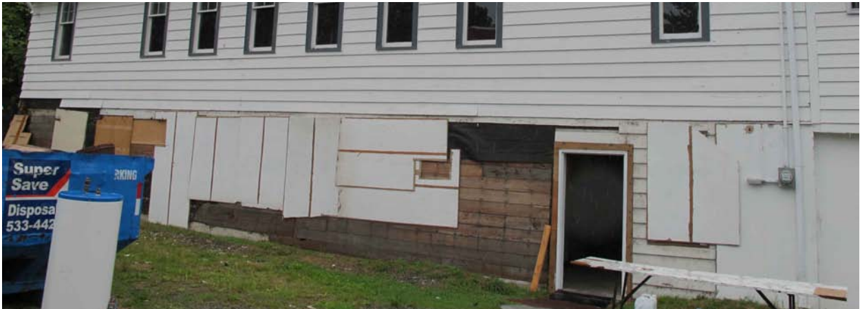
First storey wooden lapped siding
