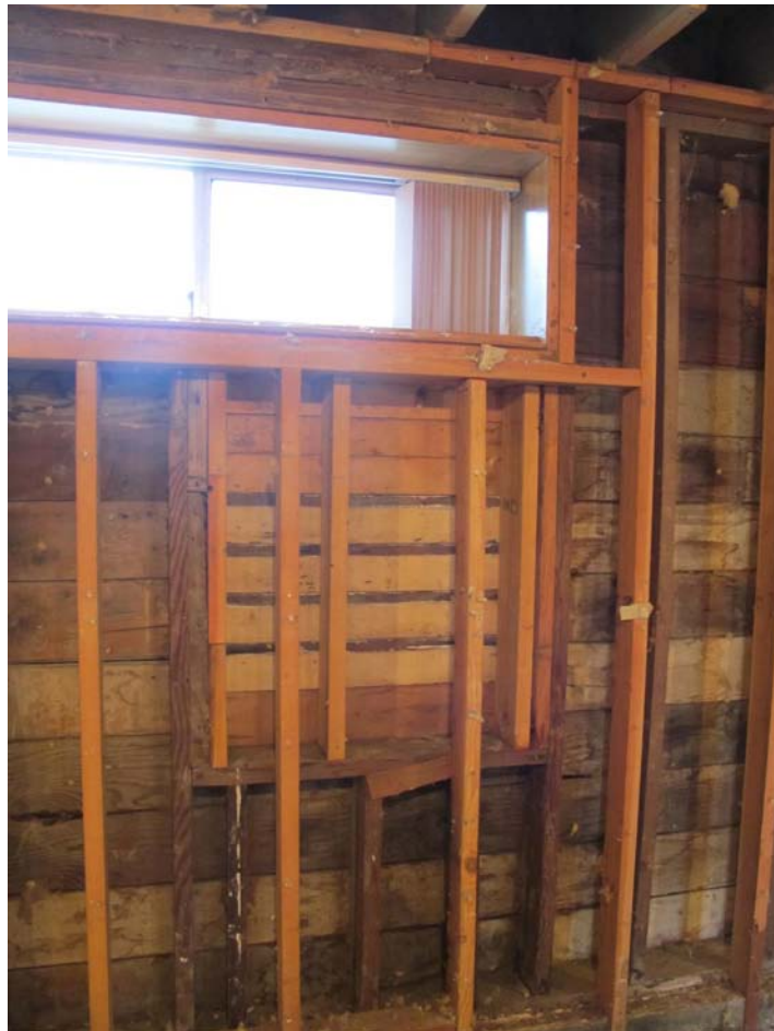
Original wooden frames on the west side of the first floor
