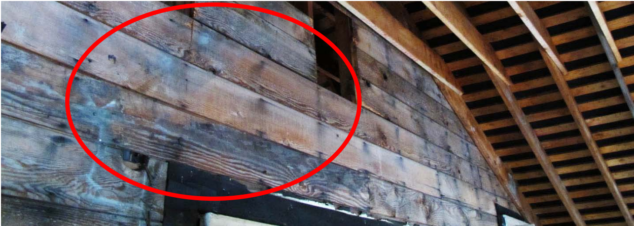
Mark showing original location of front-gabled roof above entry doors
