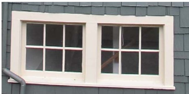
Example: Basement window
