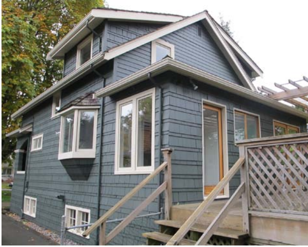
Rear (North) and East Elevations
