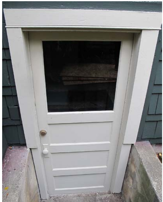
Exterior Basement Door and Hardware
