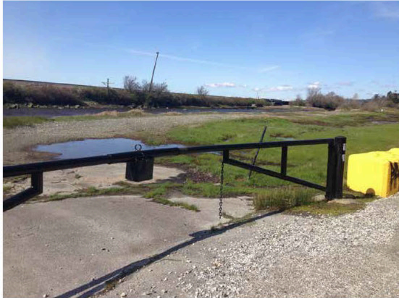
Floods to top of yellow concrete block during king tides and high water events
