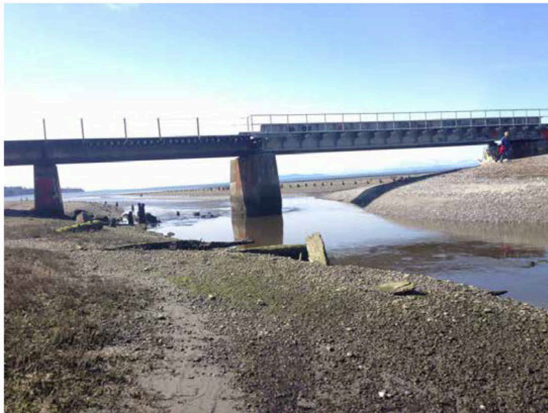
Railway Trestle, Old mill pier pilings in background
