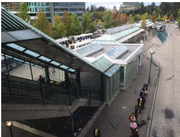
Current Day Surrey Central Exchange Looking West
