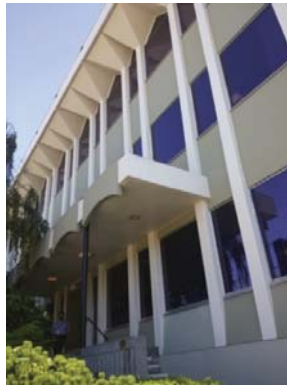
Vertical Mullions 9656 King George Blvd
