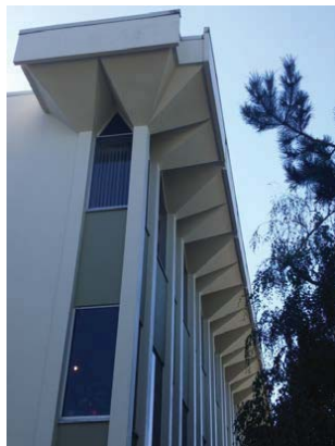
Concrete Cornice: Surrey
