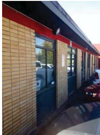
Stacked Bond on Rear Facade
