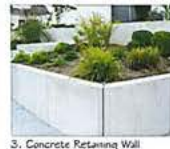
3. Concrete Retaining Wall
