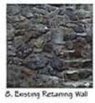
8. Existing Retaining Wall
