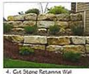
4. Cut Stone Retaining Wall
