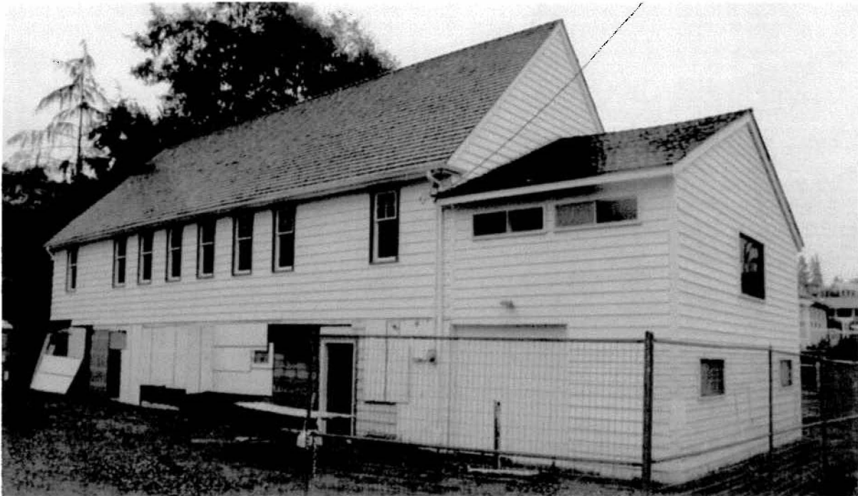
Current view of the south façade of the Seventh Day Adventist Church featuring the addition, which is to be removed
