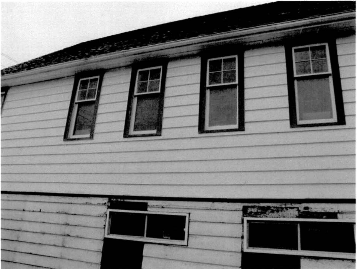
Original horizontal wooden lapped siding on the east façade
