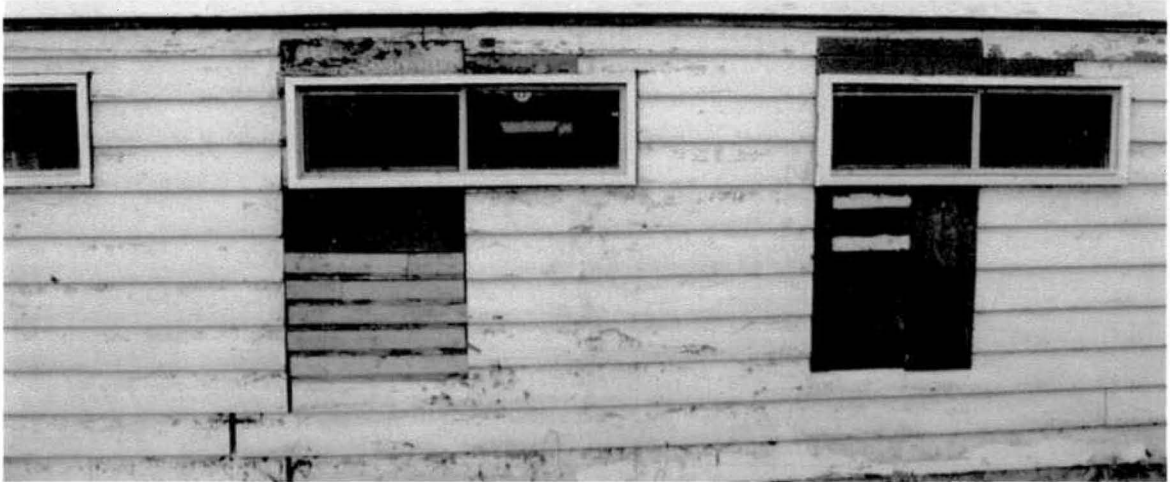
Original window outlines on the east façade of the first floor
