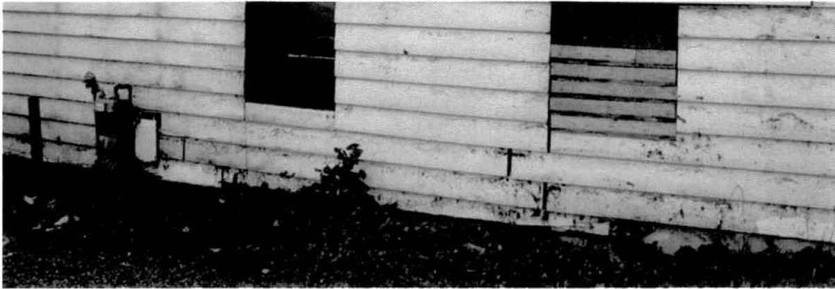
East façade of the building showing the foundation at the lower right corner
