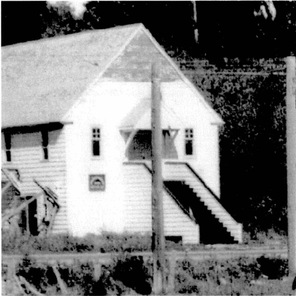
Original front entrance and steps on the south façade
