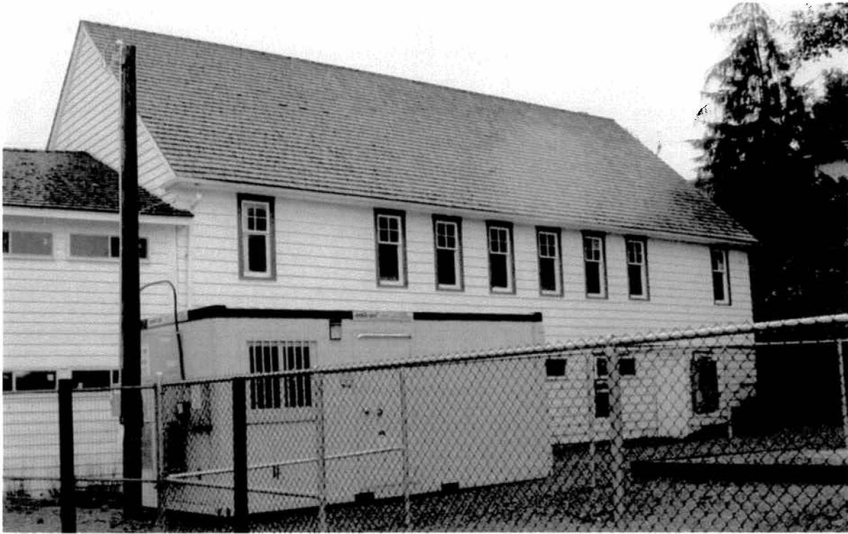
Cedar shingles on roof
