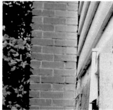
Close-up of the original chimney
