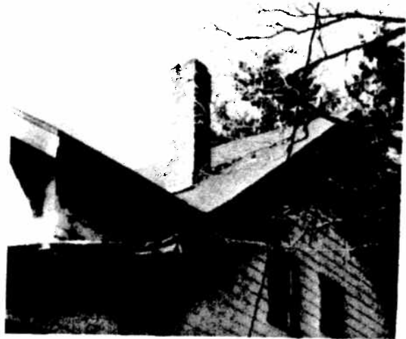
PHOTO 9: Internal Chimney (north elevation)
