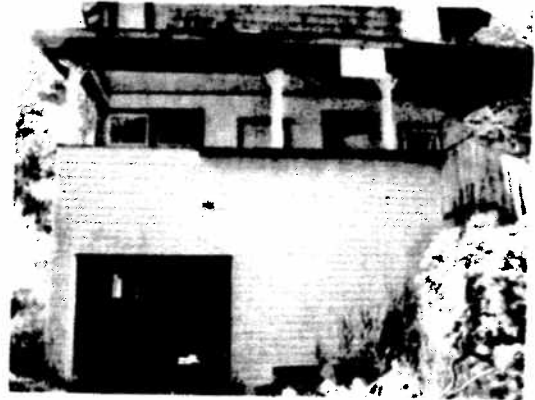
PHOTO 28: Present condition of rear porch
