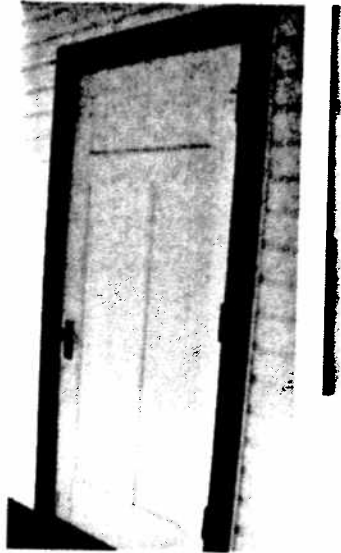
PHOTO 15: South porch Door (east elevation)
