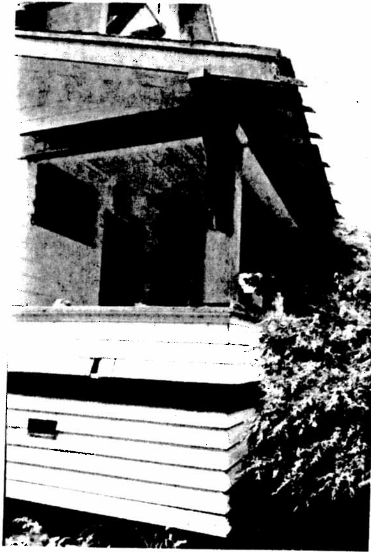
Front porch. Note notched rafters and bargeboards, ca. 1997 (City of Surrey Archives)
