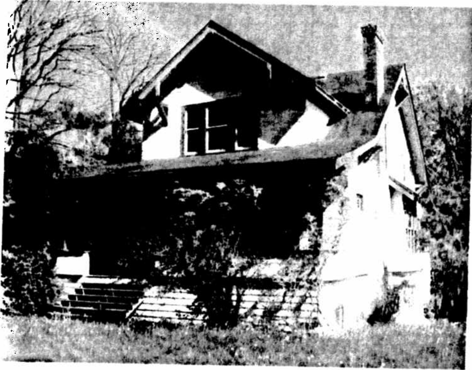
PHOTO 1: Charles Bell House (west elevation)
