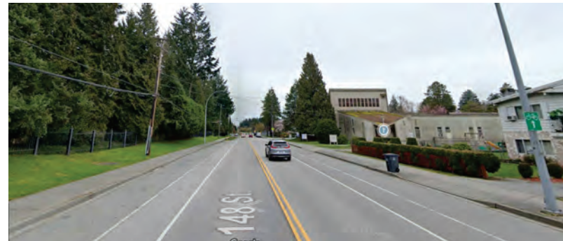
1. SOUTH -EAST VIEW OPPOSITE TO SITE (148 St)
