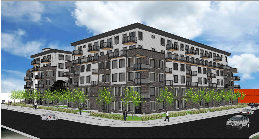
A. NORTH EAST CORNER VIEW (ALONG 103 A AVE & 149 STREET)
