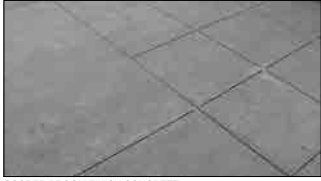
SCORED BROOM FINISH CONCRETE
