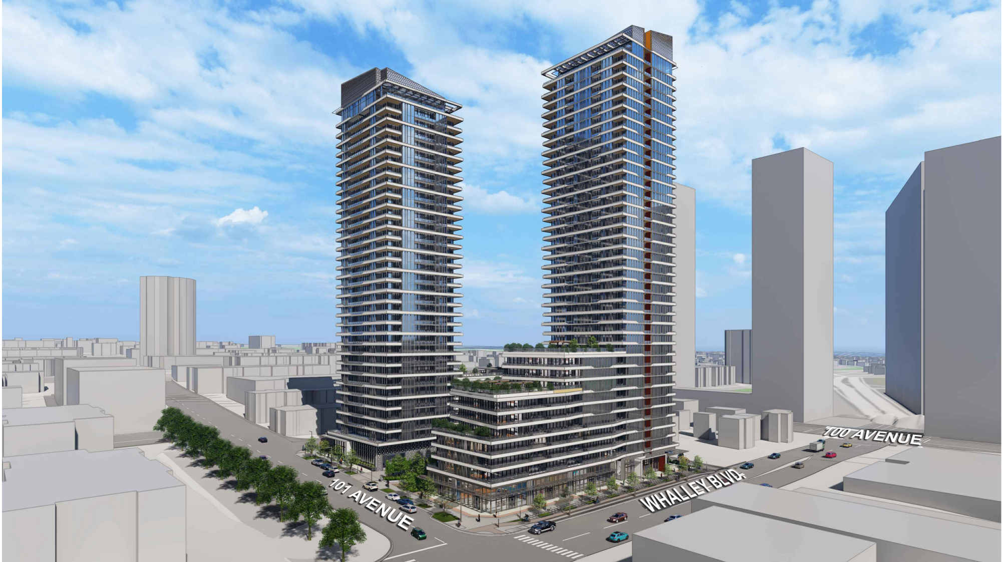
VIEW LOOKING SOUTH EAST FROM 101 AVE/WHALLEY BLVD
