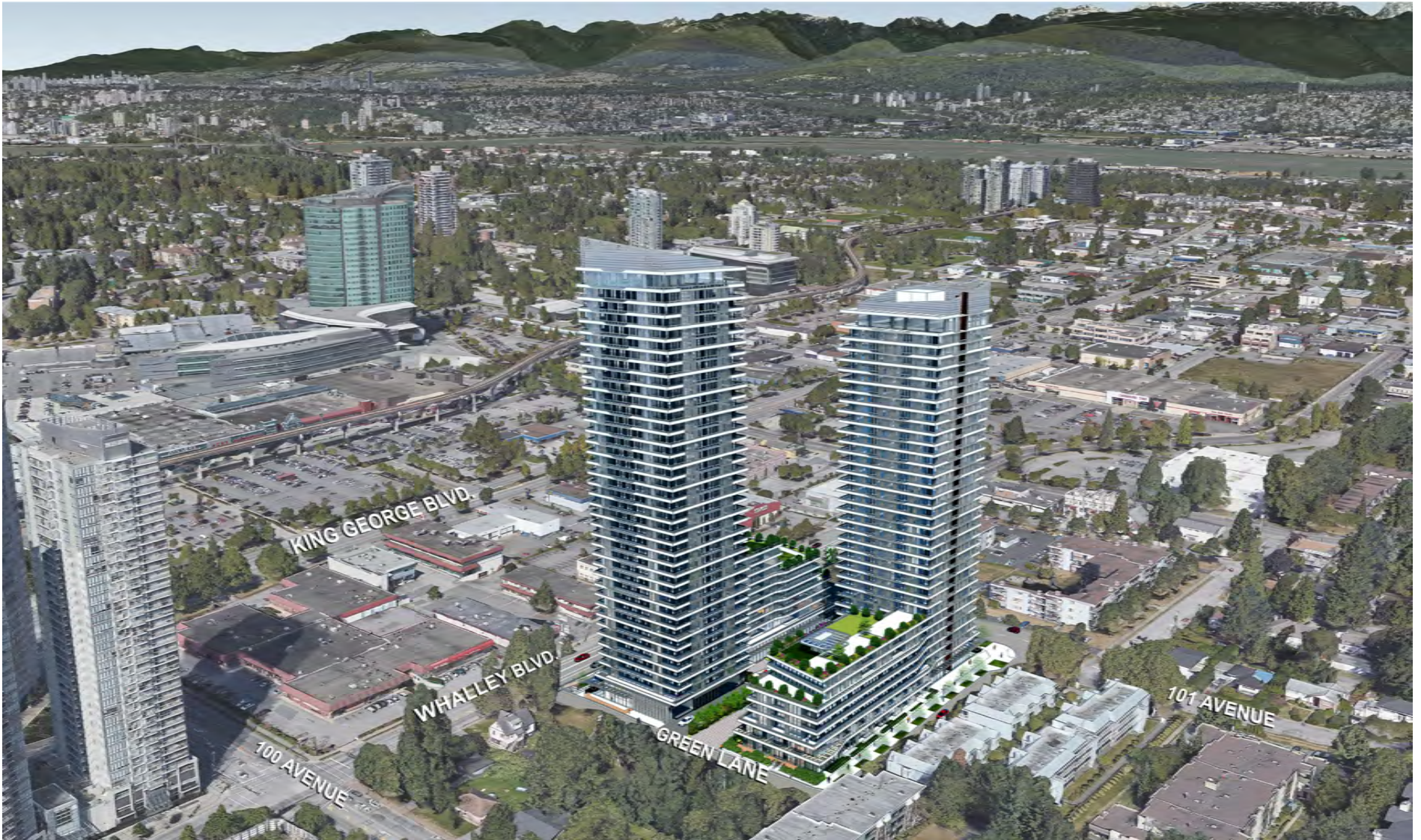
CONTEXT VIEW FACING NORTHWEST & SURREY CITY CENTRE
