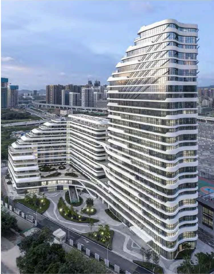
SHENZHEN METRO CHANGZHEN DEPOT COMPLEX by BLVD INTERNATIONAL
